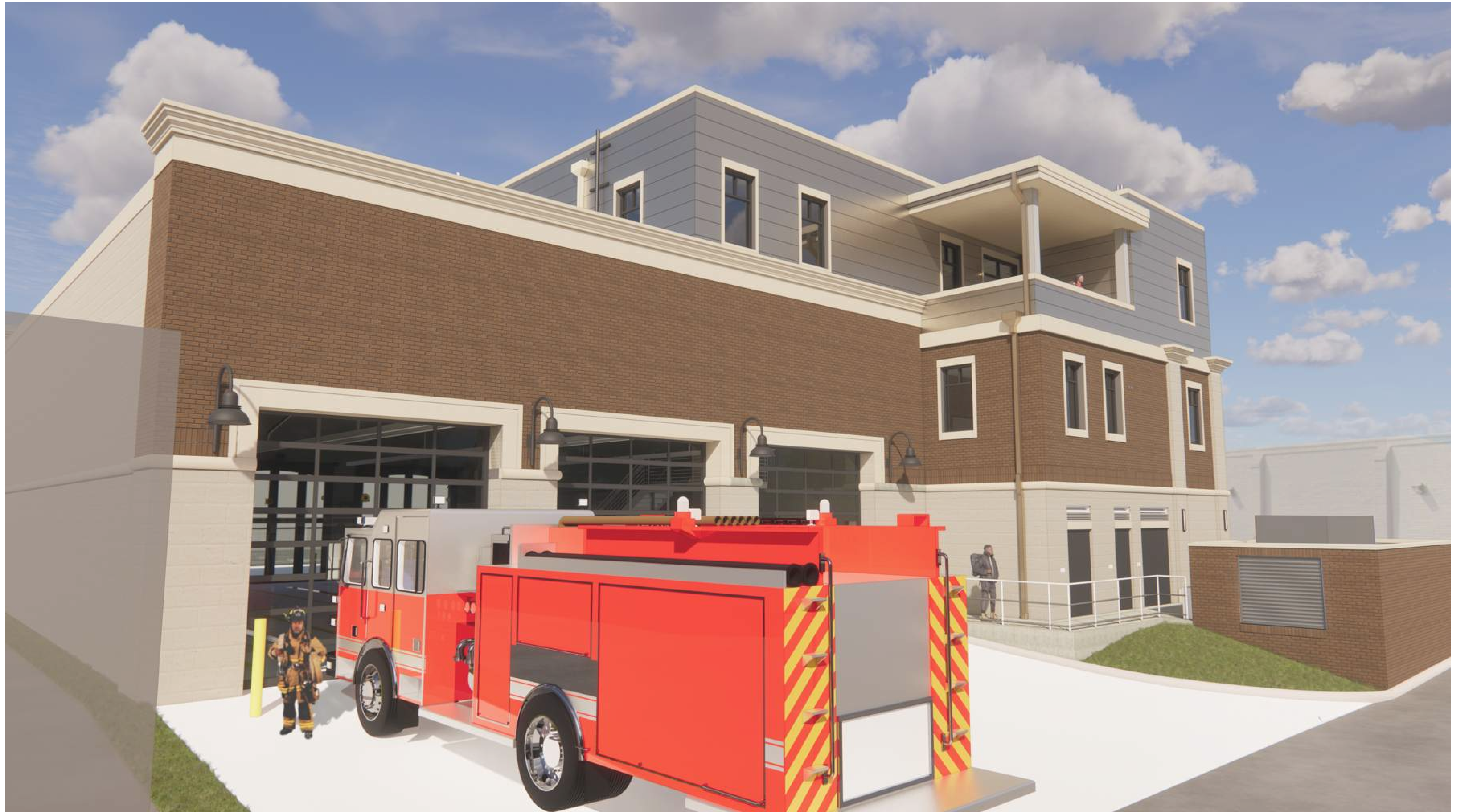
View of Rear of the Building
