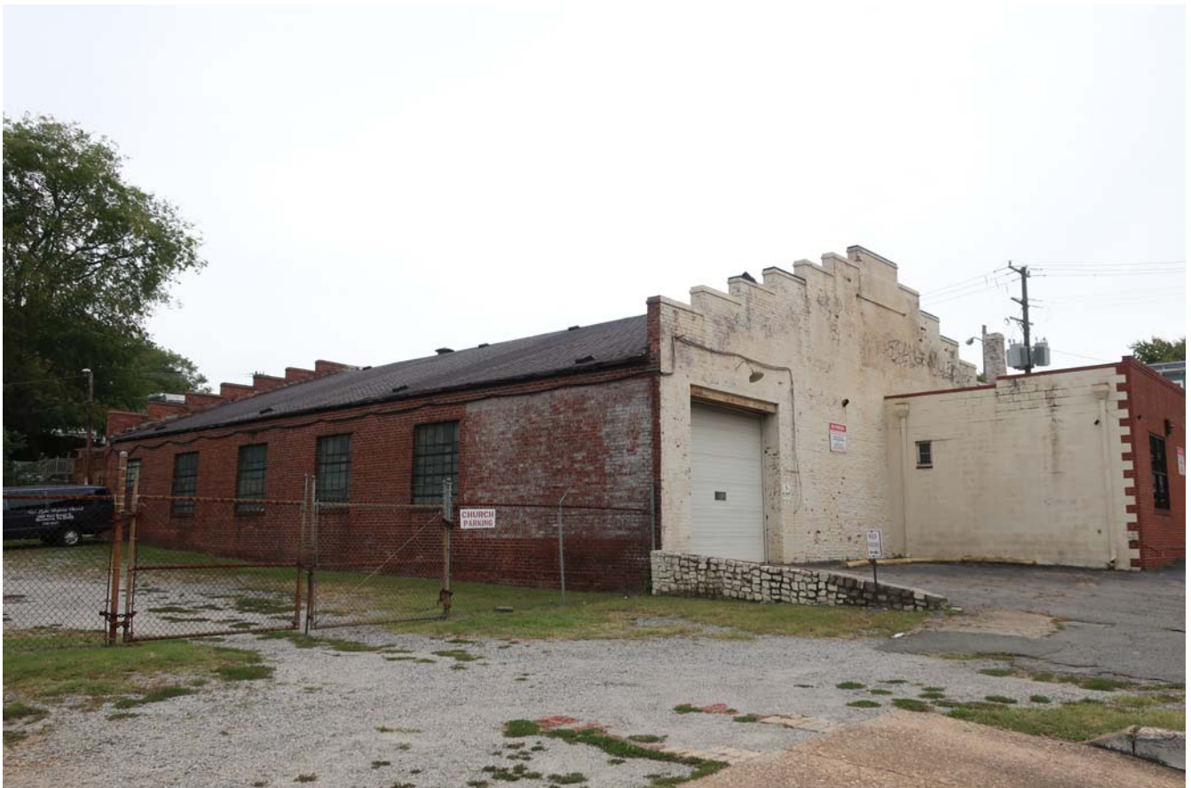
2. West side of historic garage
