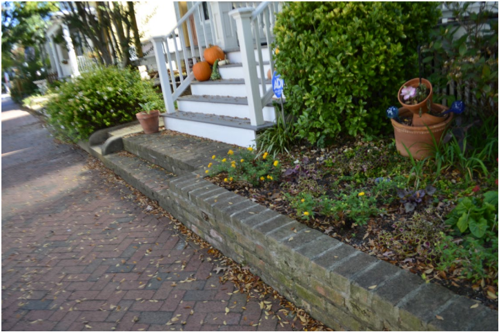
Figure 5. Low brick wall west of 311 North 32 nd Street.
