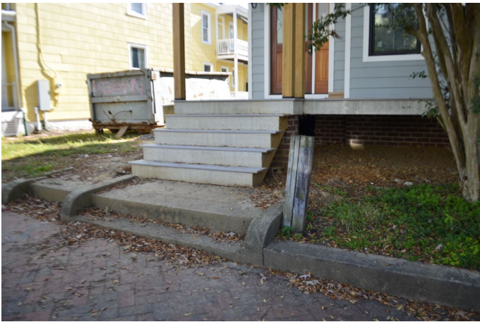
Figure 3. The staircase of the new house at 313 North 32 nd Street does not line up with the historic concrete step and curb.
