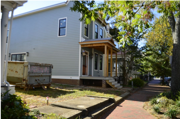
Figure 6. Extant concrete curb and concrete steps, along the east side of North 32 nd Street.
