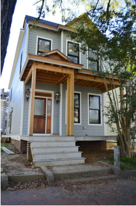
Figure 1. Façade, west side of 313 North 32 nd Street.
