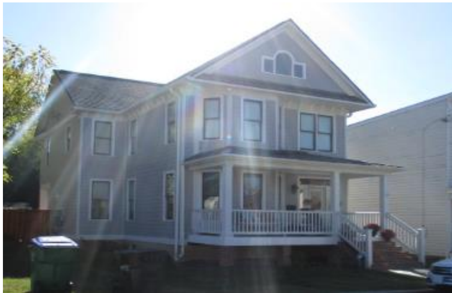
Figure 3: CAR approved dwelling at 2317 Carrington Street
