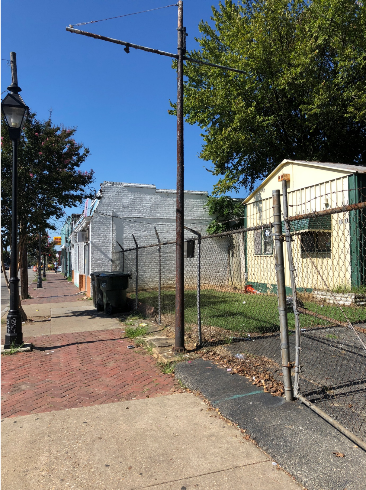
Image 2 – View of curb entry, existing structure, existing chain link fence with barbed wire, and existing pole to be removed.
