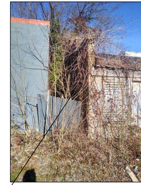
REAR OF PROPERTY (SOLID BRICK WALL)
