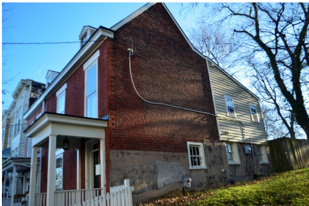
Figure 5. View of the neighboring two-story addition at 617 North 26 th Street.
