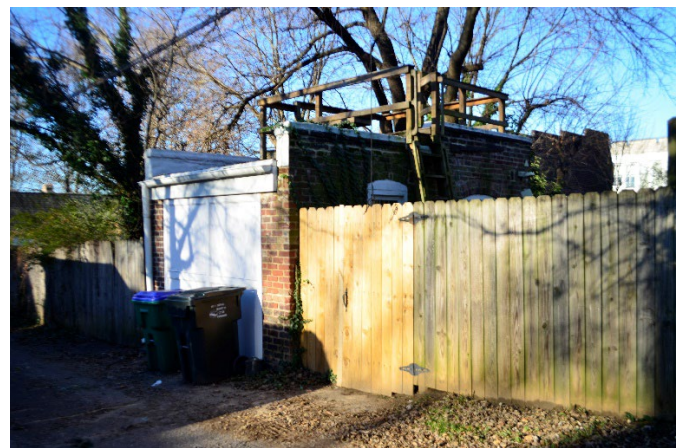
Figure 2. Historic rear garage at 611 North 26 th Street.
