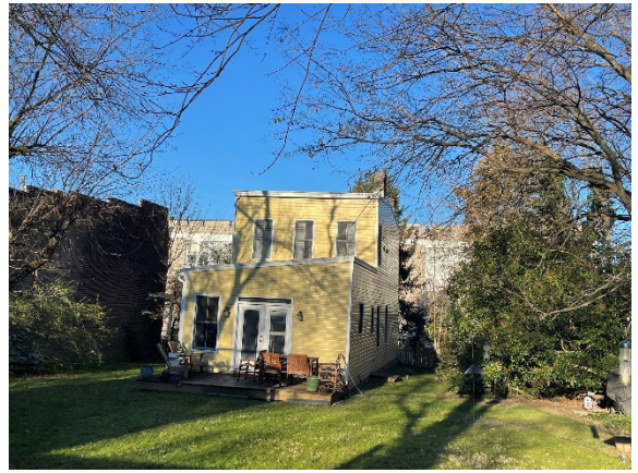
Figure 4. View of the rear of 611 North 26 th Street from the public alley.
