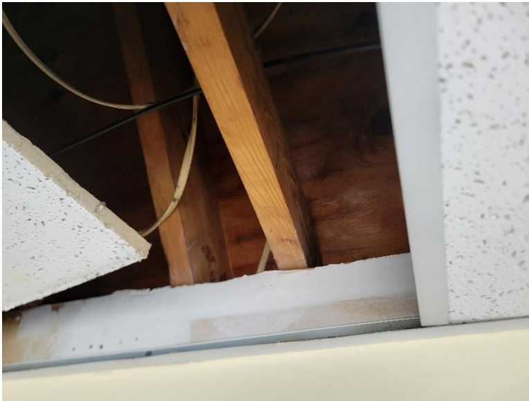
Valet Booth – ceiling and framing showing plywood sheathing
