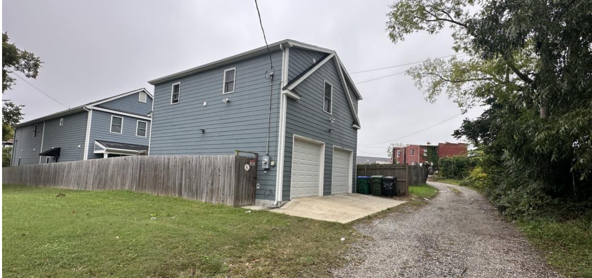
Figure 3: Picture of accessory building at 2413 Carrington fronting the rear alley
