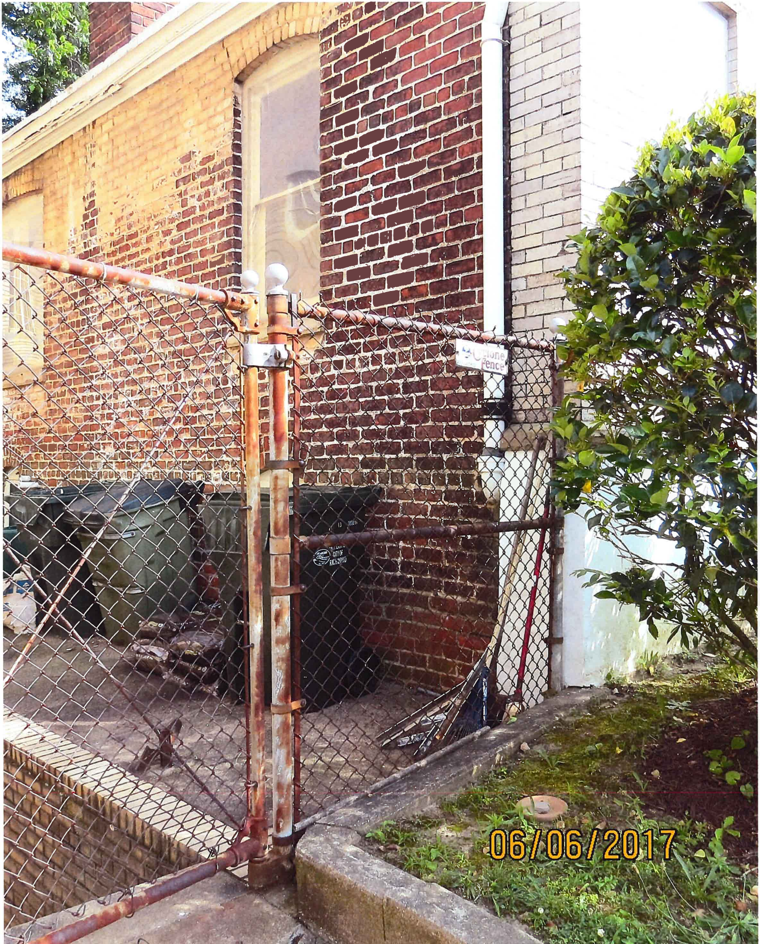
entrance from side walk
