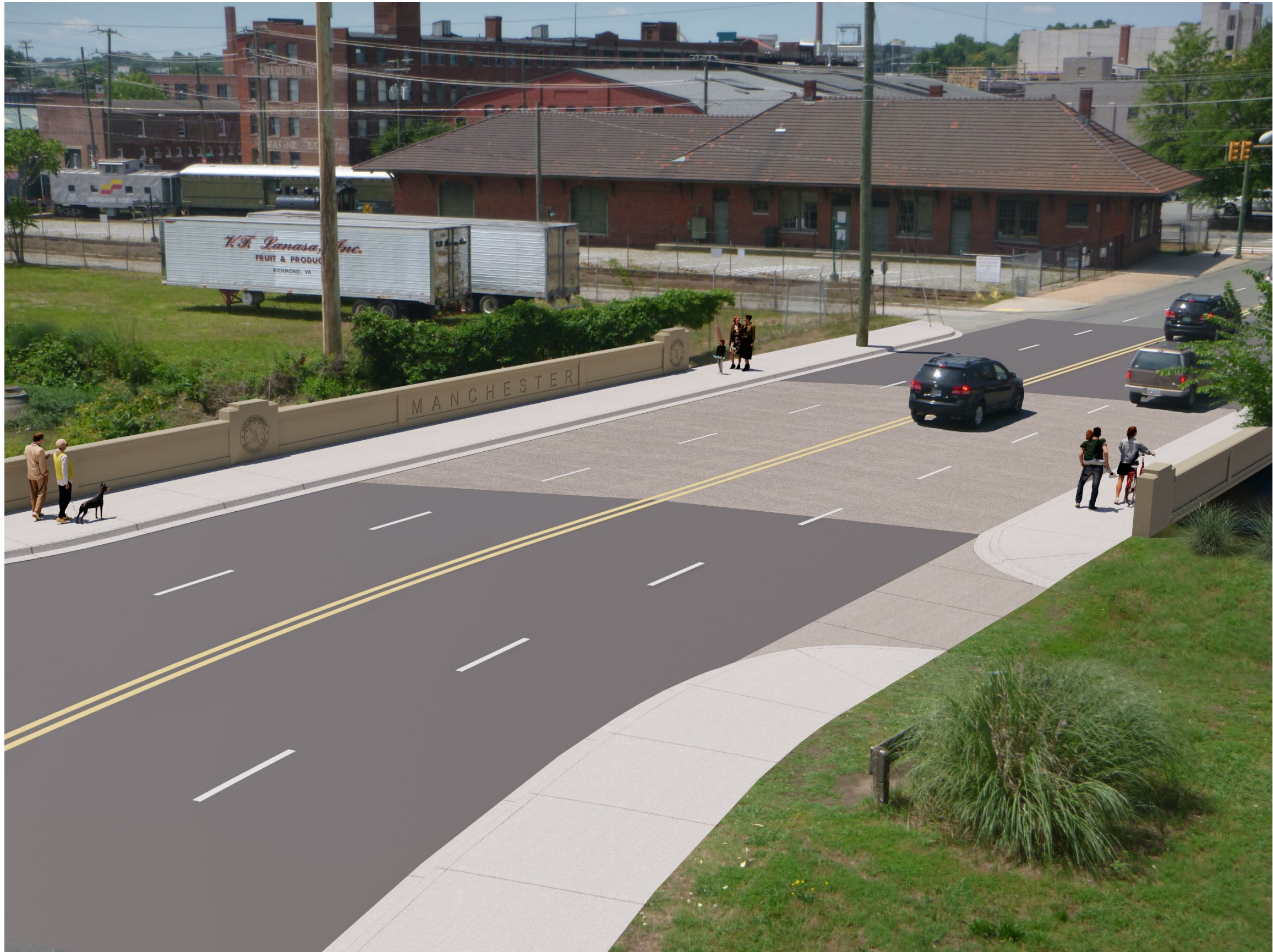
Figure 1 - View from Floodwall
