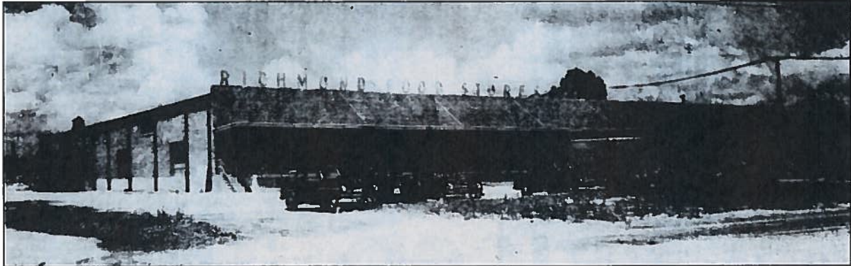
Figure 1: The Richmond Food Stores building located at 2522 Hermitage Road in 1949. (RTD 6/29/1949)
