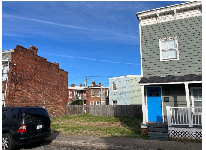
Figure 4. Subject lot at 2316-2318 Burton Street.
