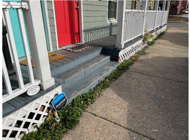
Figure 6. Steps on the front porch of 2320-2326 Burton Street are set back into the porch floor, rather than encroaching into the right-of-way.
