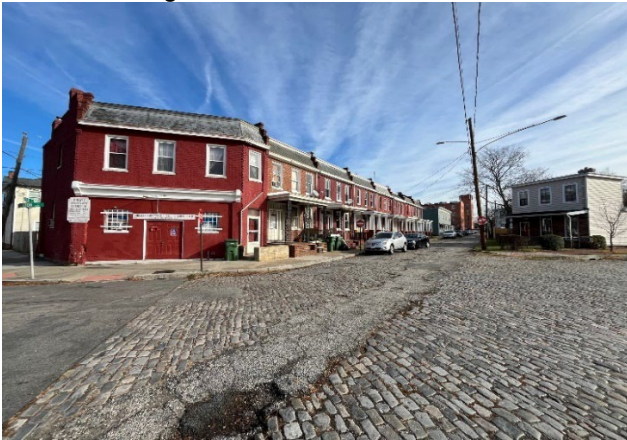
Figure 7. Block context. Intersection of Burton and Tulip Streets looking east down Burton Street.
