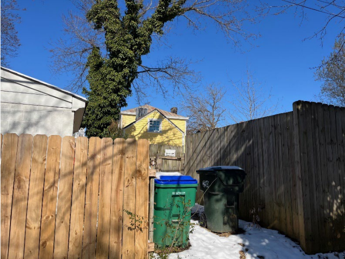
Figure 5. View of existing rear addition from the rear alley.
