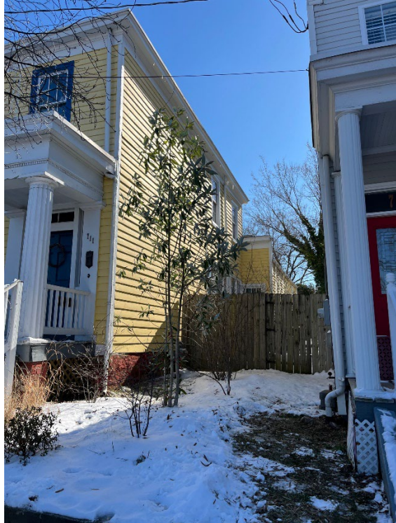
Figure 2. View of existing rear addition from North 26 th Street.
