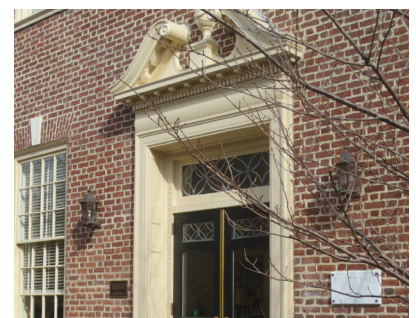
View of Ellet Hall Entry
