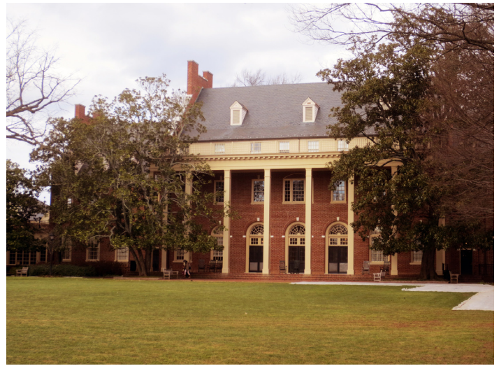
View of Portico at Bacot Hall
