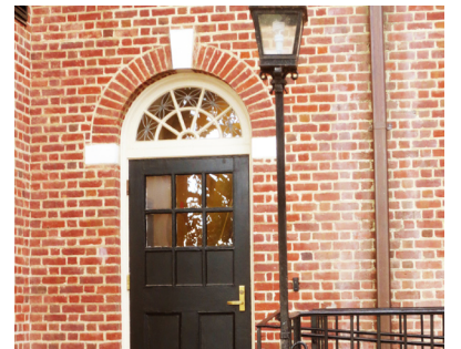
View of Entry Detail
