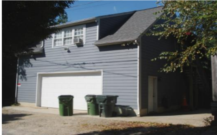
Figure 2: Image of the existing detached garage on the Property
