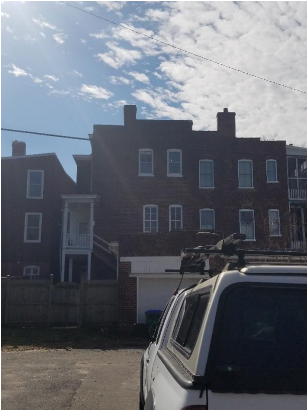
Figure 5. 3420 E. Broad Street, facade and existing rear stairs.
