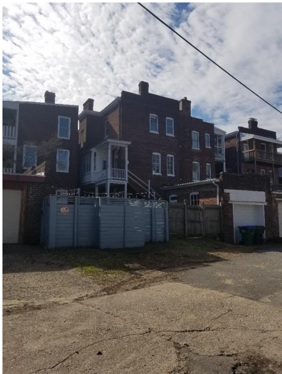
Figure 4. 3420 E. Broad Street, rear elevation.
