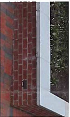
BRICK SEAT WALL WITH CONCRETE CAP
