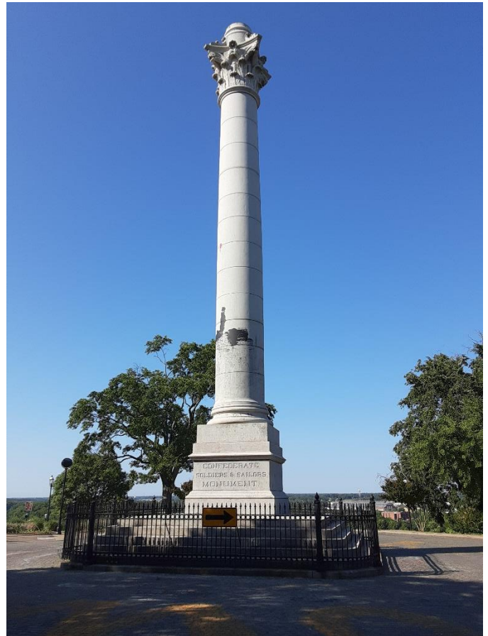
Figure 2. Confederate Soldiers and Sailors Monument, current condition.
