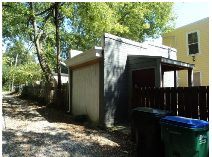
Figure 4. Nearby historic garage
