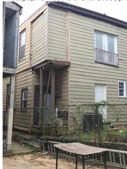
Photograph 3. 705 North Street, rear, current conditions.
