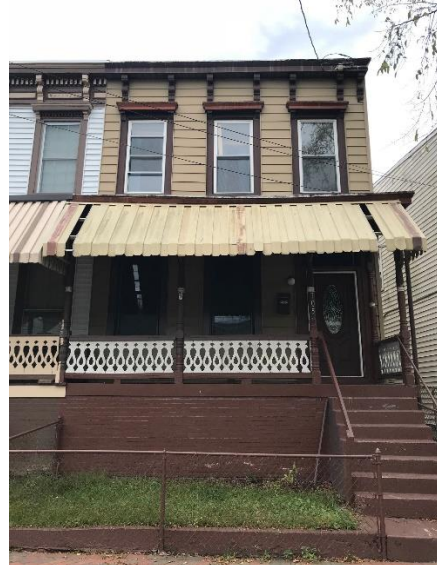
Photograph 2. 705 North 21st Street, present.
