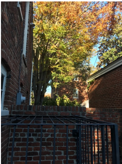
Figure 3. Rear elevation of structure.
