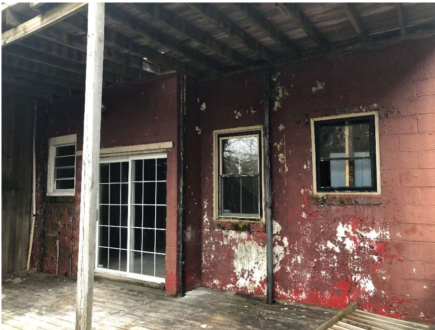
Cinder block addition
