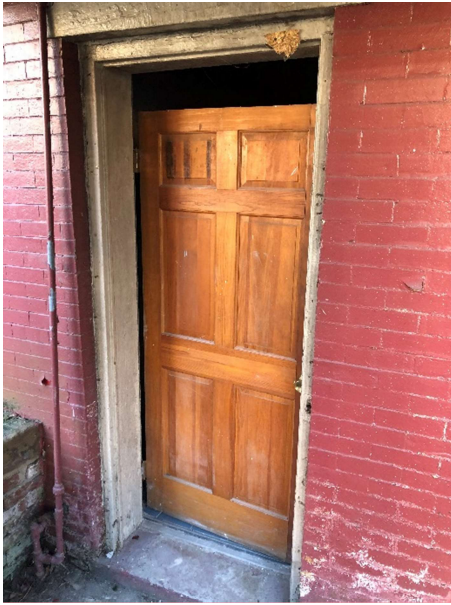
Current front basement door
