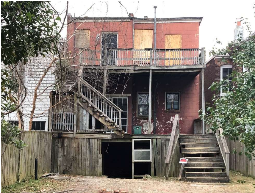
Rear of property, showing 1947 cinder block addition and deck.
