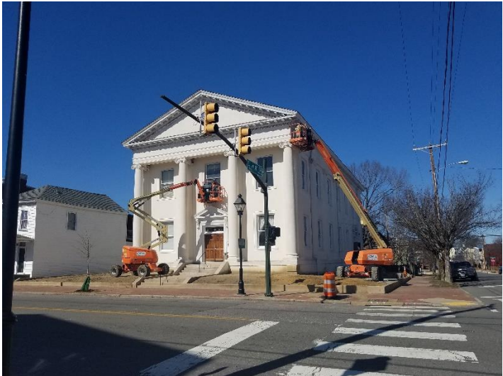
Figure 1. 520 N. 25th Street.
