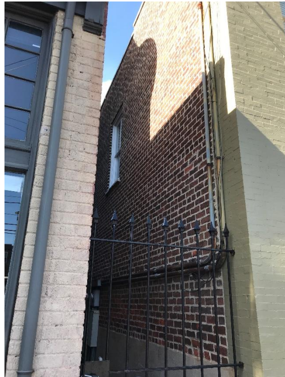
Figure 2. View of side elevation from North 26th Street.
