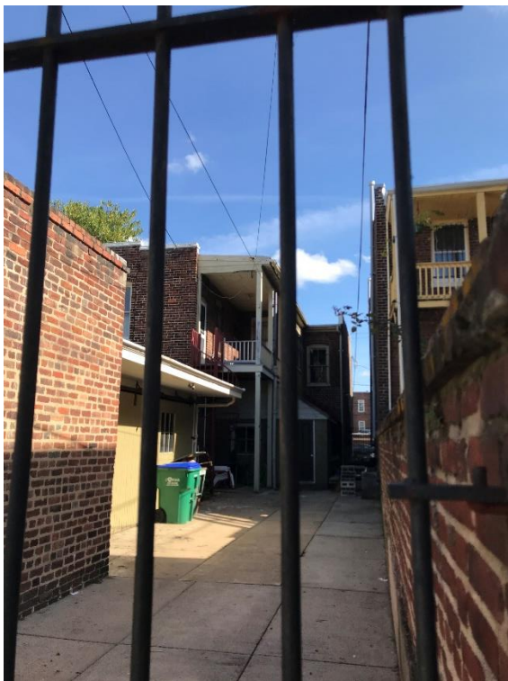
Figure 1. View of rear from alley.
