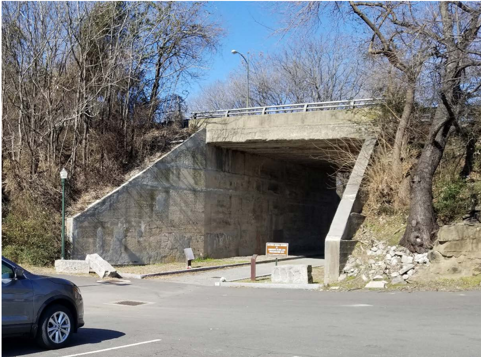
Broad St over Abandoned RR Spur – Existing Condition
