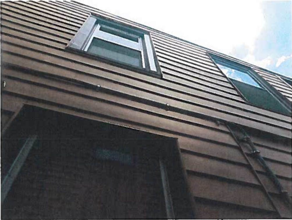
- Upper level Windows (replaced with wood).
