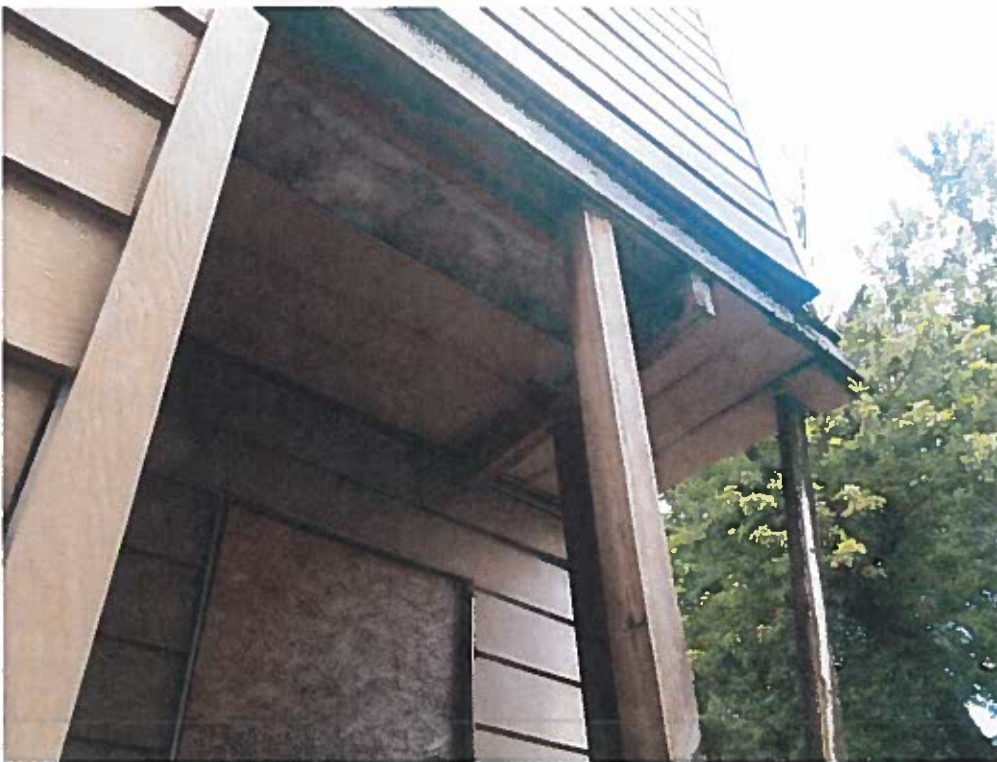
- Non-code supports (close in area to fully support upper level).
