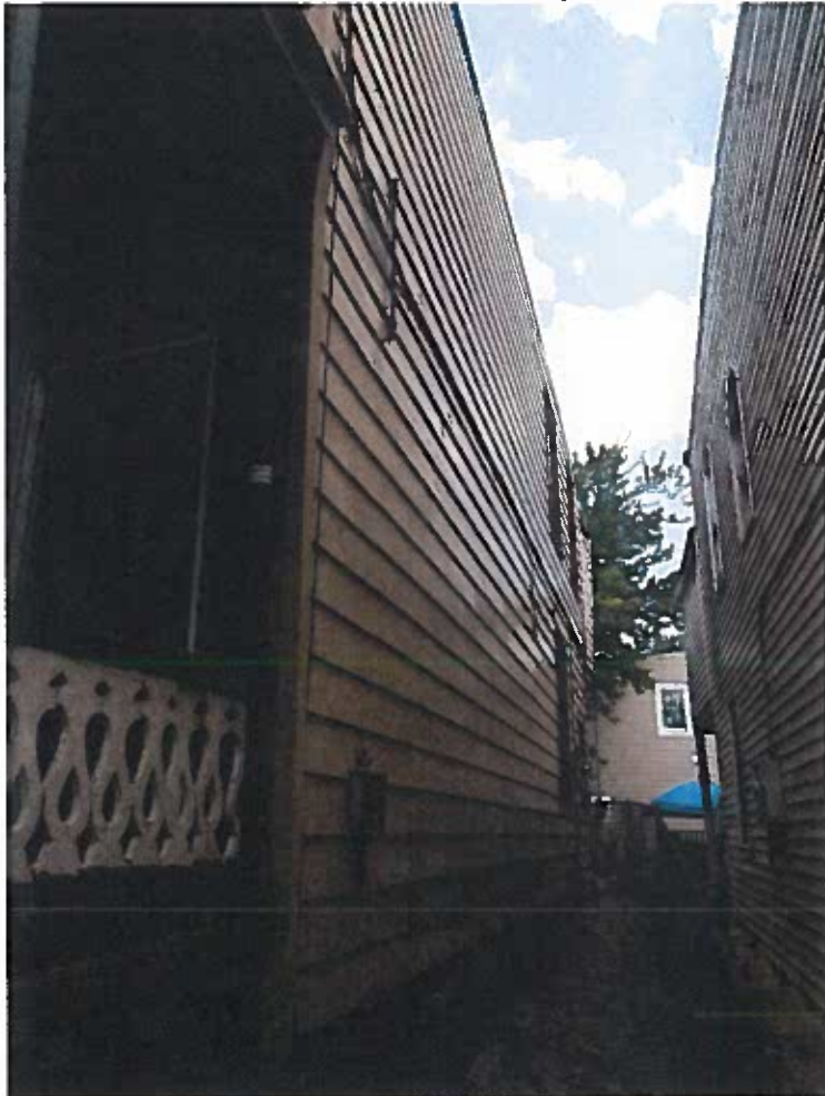
- Siding (replace with smooth hardie plank.)
