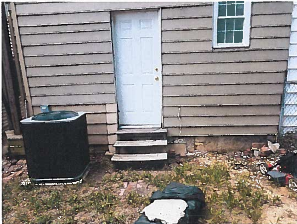
- Back door (replace outdoor unit, install on the roof; add concrete patio).
