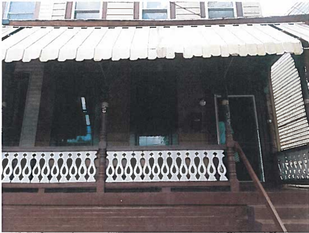
-Front Porch (remove awning, replace spindles with Richmond Rail)
