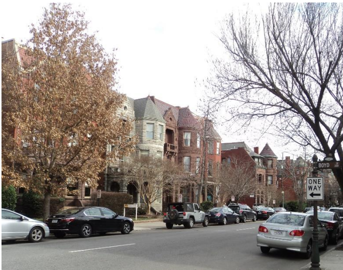
Figure 3. North side of West Franklin Street
