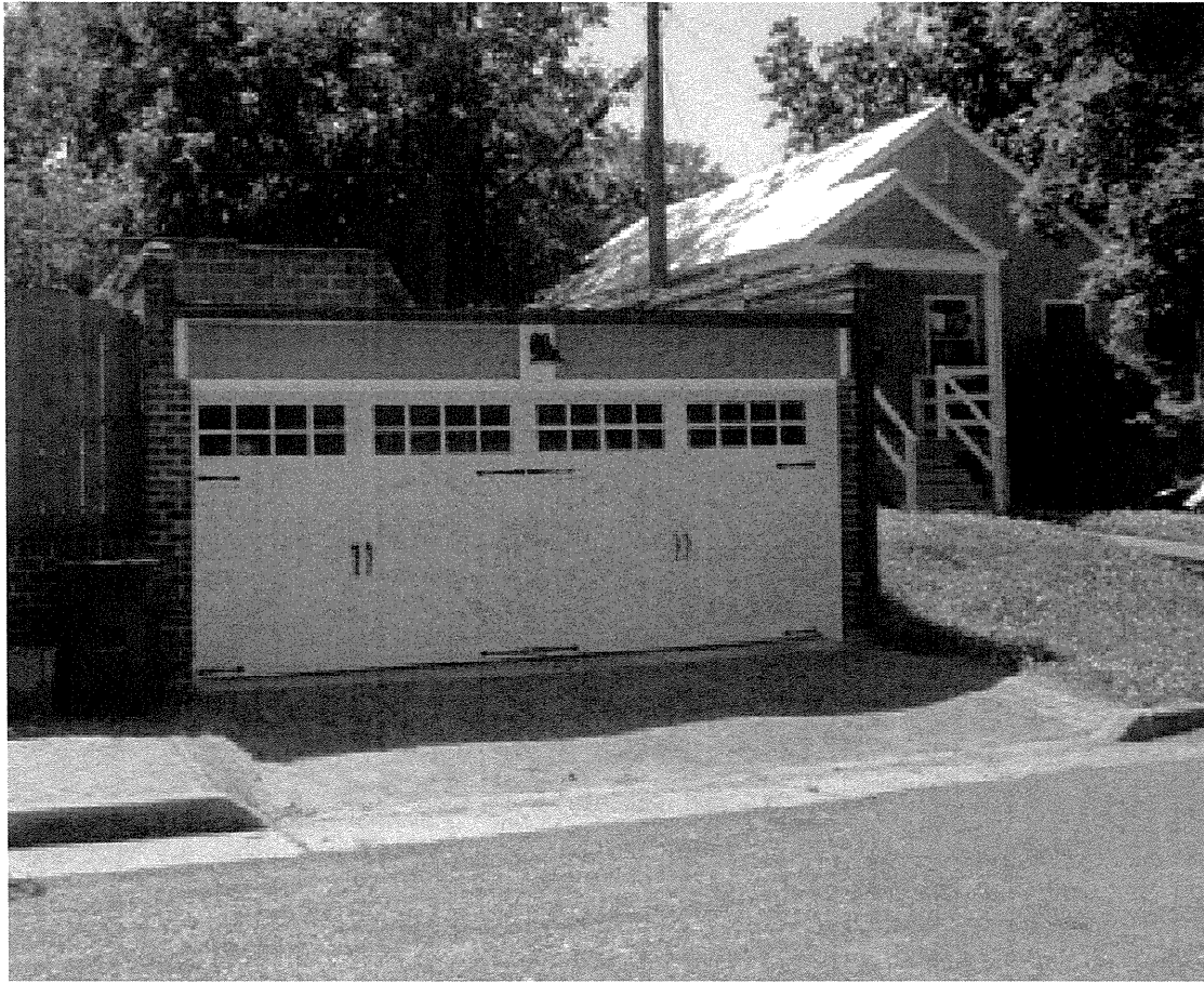
31st view - new curb cut built to property line
