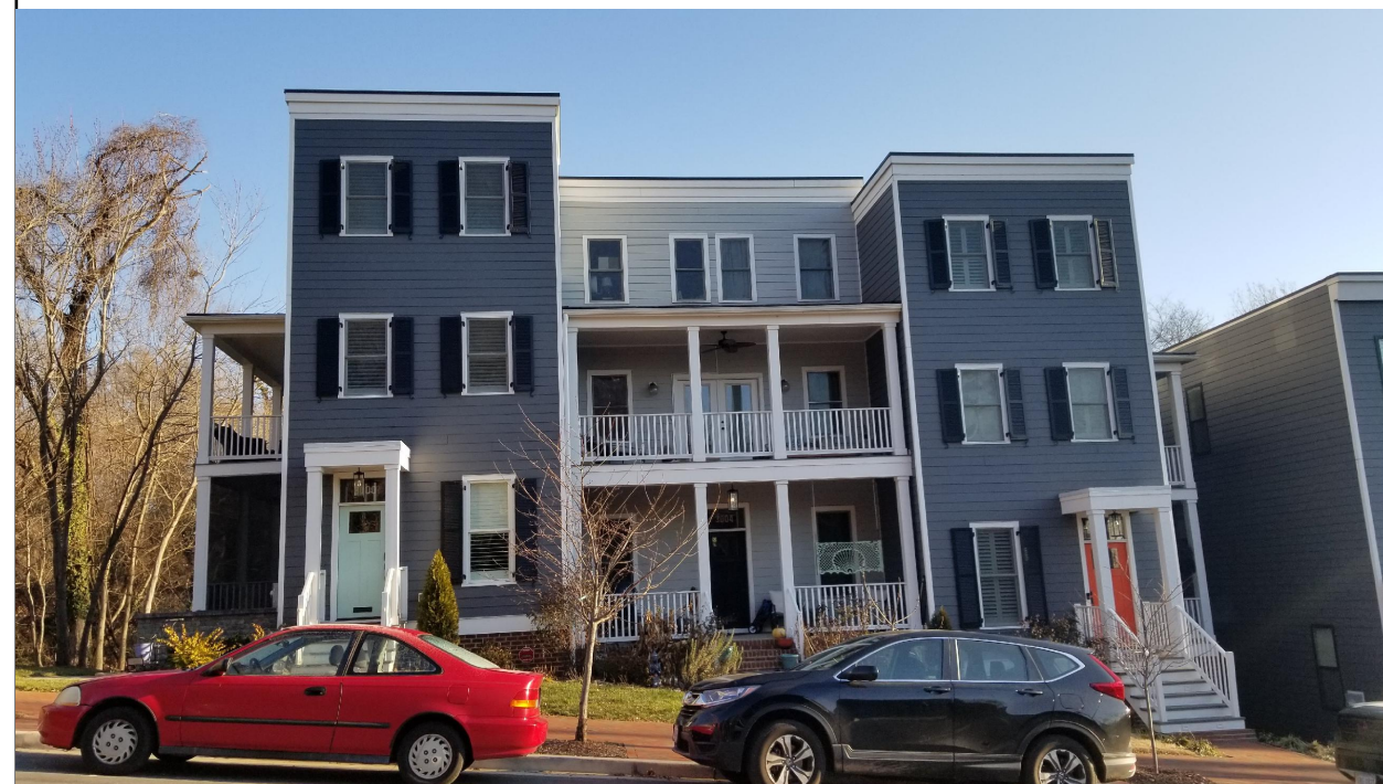
3000-3006 E. FRANKLIN ST. HOUSES
