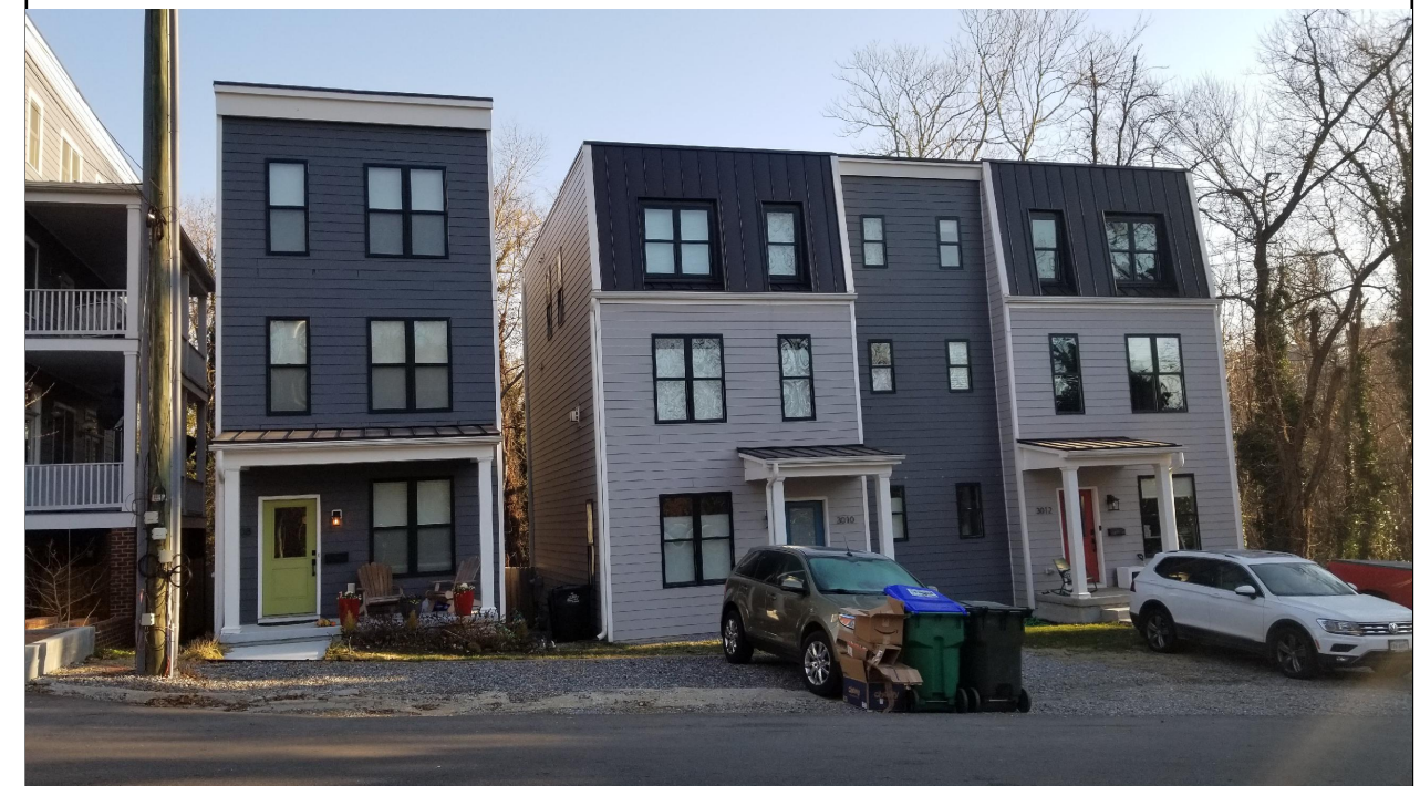
3008-3012 E. FRANKLIN ST. HOUSES
