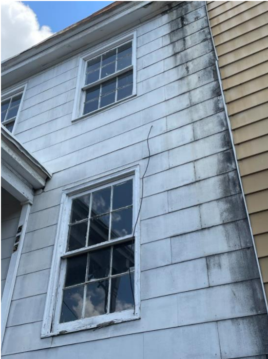
Figure 5. Current condition of windows
