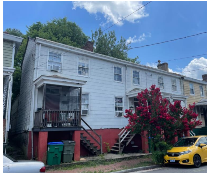
Figure 2. Front façade of 3 attached homes
