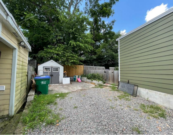
Figure 11. Rear view from alley of another property
