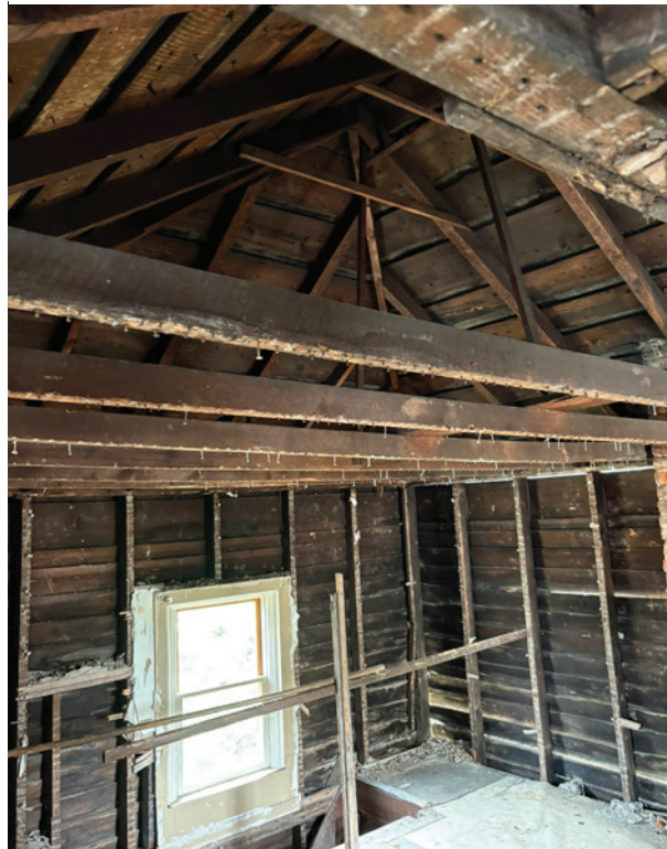
View of non-original window and original roof structure that will be maintained and relocated upwards
