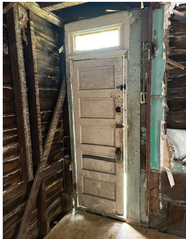
View of door and transom - the door appears to be a replacement. Project proposes removal of both for structural reasons.
