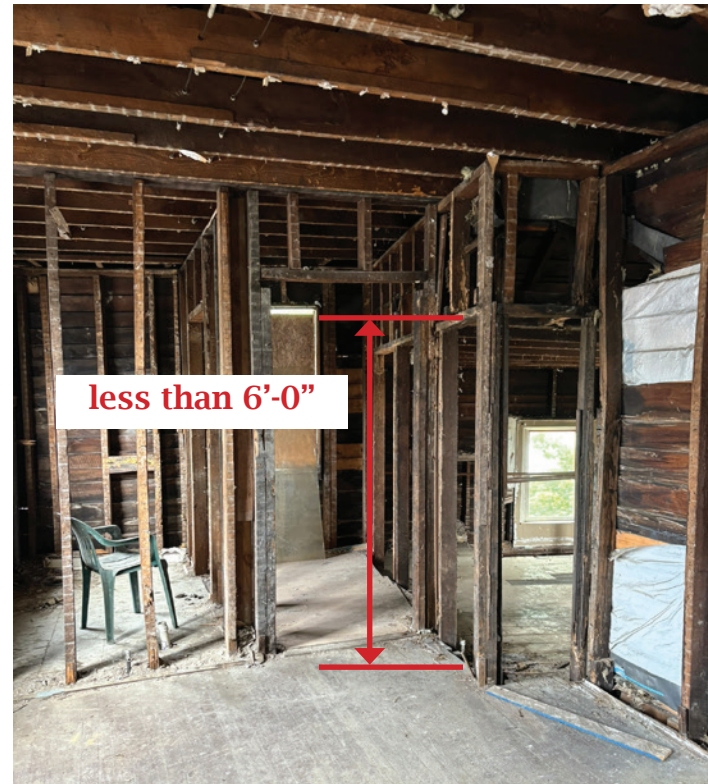
View of second floor and low headroom at intersection of volume 1 and volume 3
