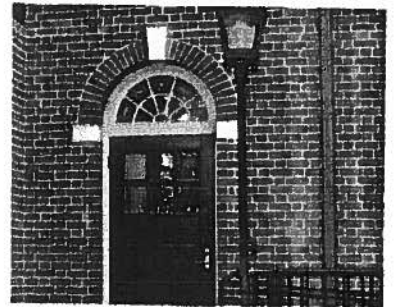
View of Entry Detail
