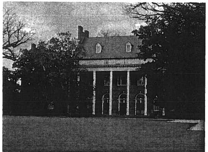
View of Portico at Bacot Hall
