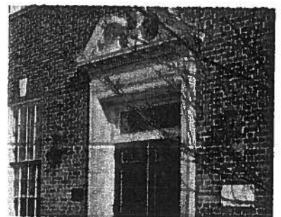
View of Ellet Hall Entry
