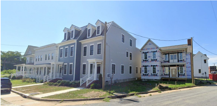
Figure 7. Several examples on new construction in the immediate area. Carrington & Pink Streets.
