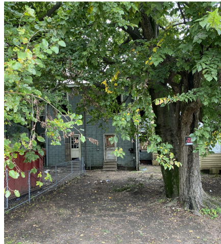
REAR ELEVATION - AS SEEN FROM PUBLIC ROW (alley behind)
