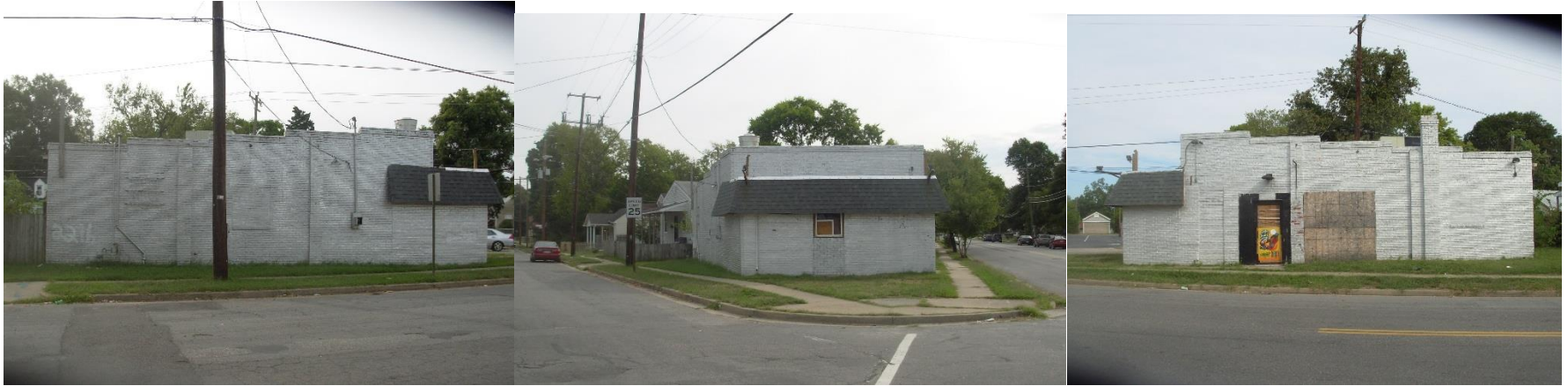
2216 Keswick Ave – Commercial Structure
