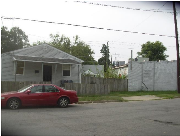
2216 Keswick Ave – Residential & Commercial Structures
