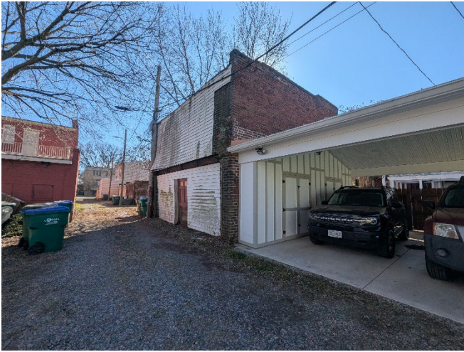
Figure 6: subject two-story carriage house
