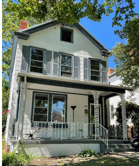
Figure 8. View of 600 West 20 th Street.
