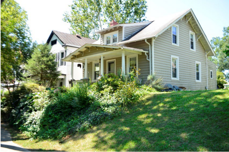
Figure 7. View of 602 and 604 West 20 th Street.
