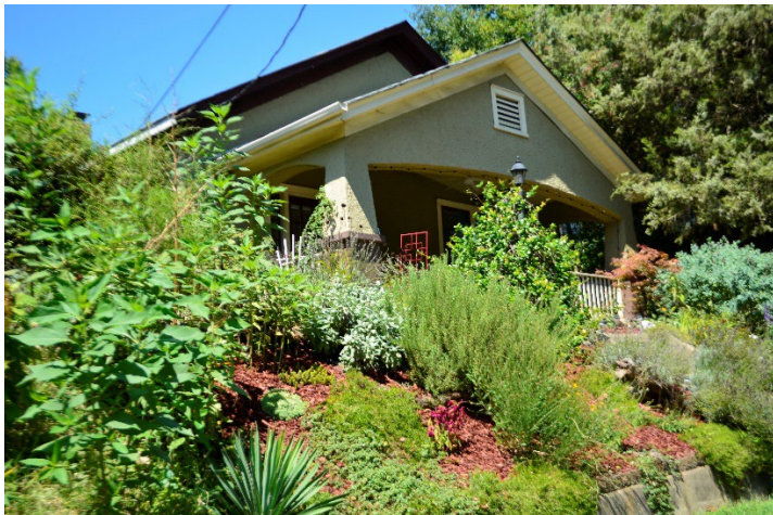
Figure 5. View of 614 West 20 th Street
