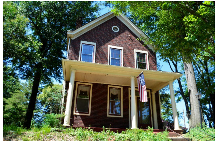
Figure 2. View of 618 West 20 th Street. The new dwelling will be located on the south portion of this lot, which is the overgrown section in the left side of the photograph.
