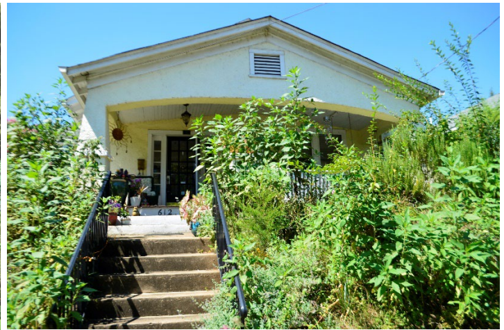
Figure 6. View of 612 West 20 th Street.
