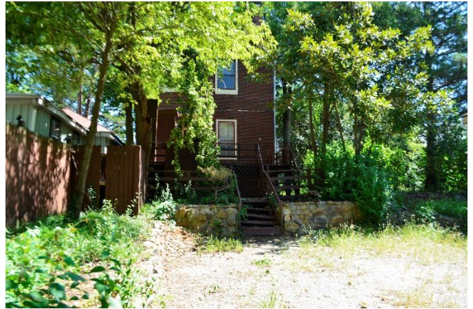
Figure 12. Rear view of 618 West 20 th Street.
