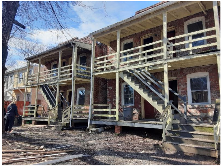
Figure 4. 311-313 N. 33rd Street, rear elevation porches.
