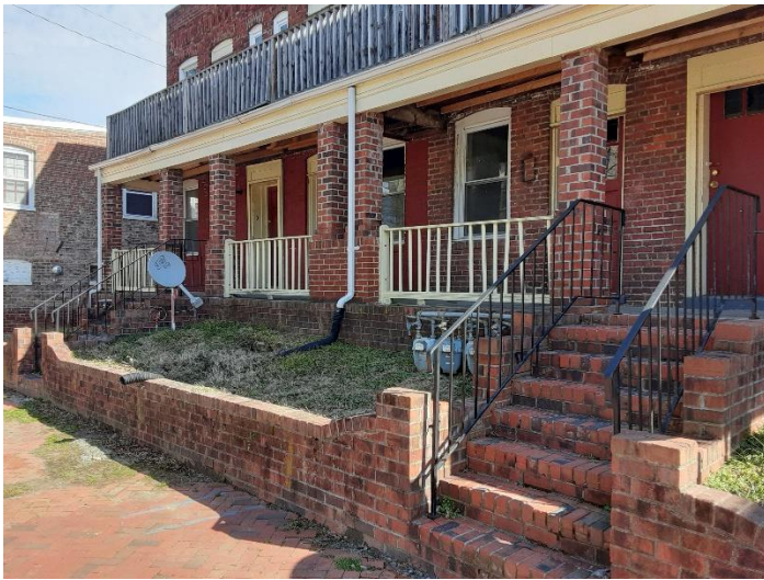
Figure 3. 311-313 N. 33rd Street, facade railing details.
