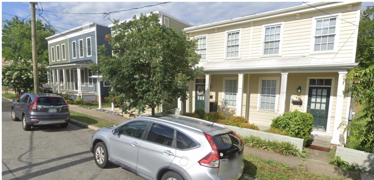
Figure 5: CAR approved dwellings along Pink Street with TPO roofing material and mansard roof form
