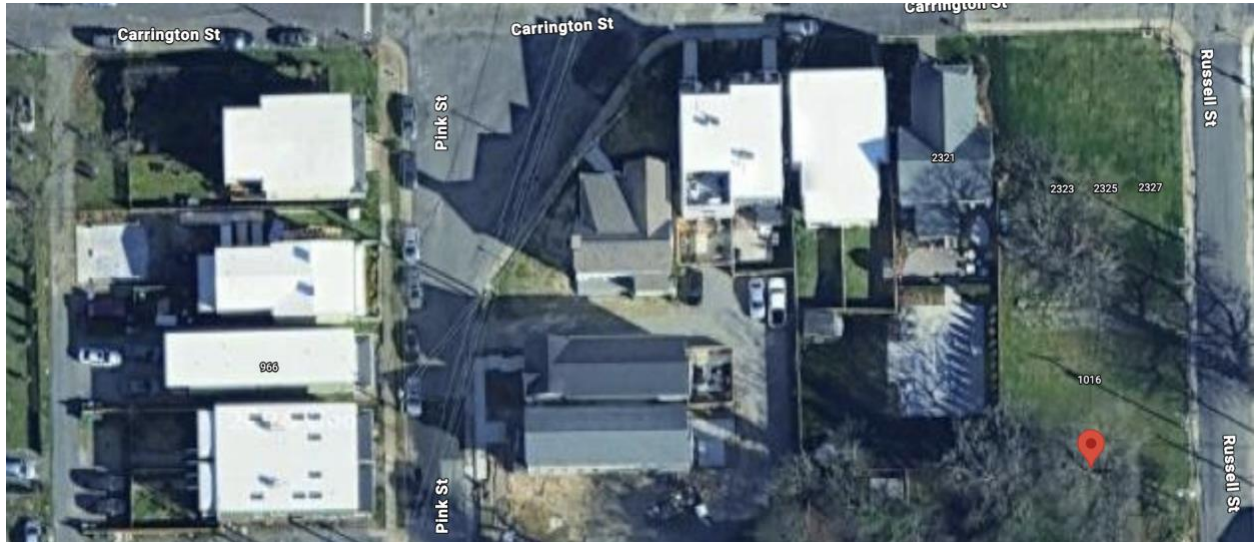
Figure 4: CAR approved dwellings along Pink Street with TPO roofing material and mansard roof form
