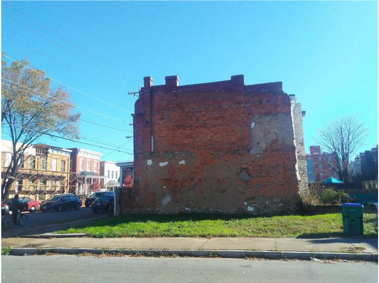
Figure 2 2301 Venable looking East from Tulip St
