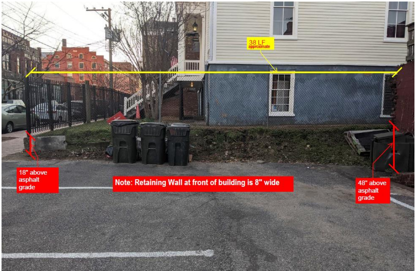
Figure 3. Existing conditions of West elevation of Masonic Hall.
