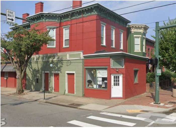
Figure 4: While not in the Union Hill historic district, this mixed-use building is an example of a protruding corner commercial storefront
