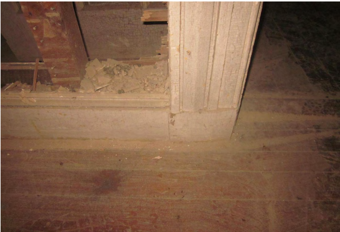
Photo 9.7 Interior Woodwork, plinth block and two member baseboard at 1 st Floor
