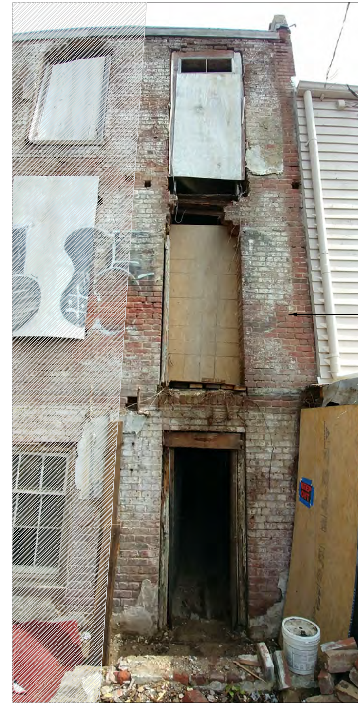
SECTION TO BE REPOINTED D5 NTS
