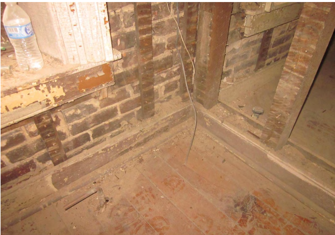
Photo 9.9 Interior Woodwork, beaded baseboard at 2 nd Floor
