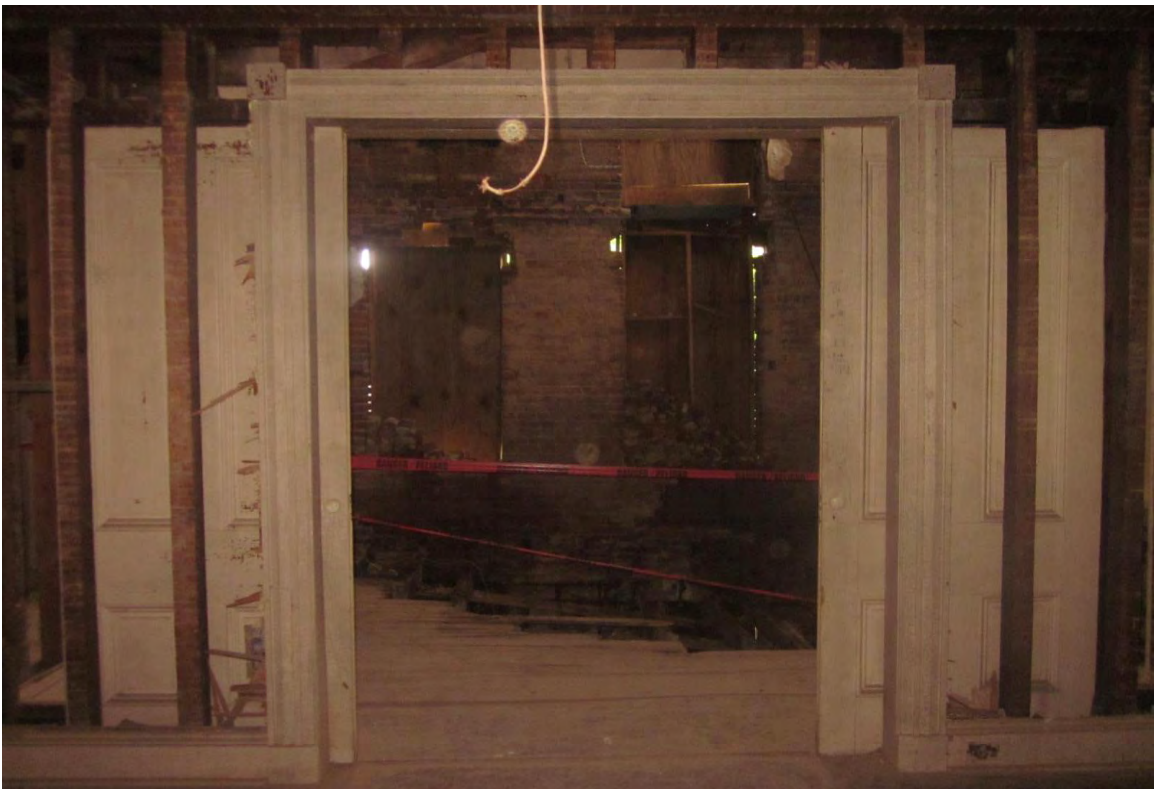
Photo 9.5 Interior Woodwork; Interior Doors, original pocket doors between Room 3 and Room 4 to remain
