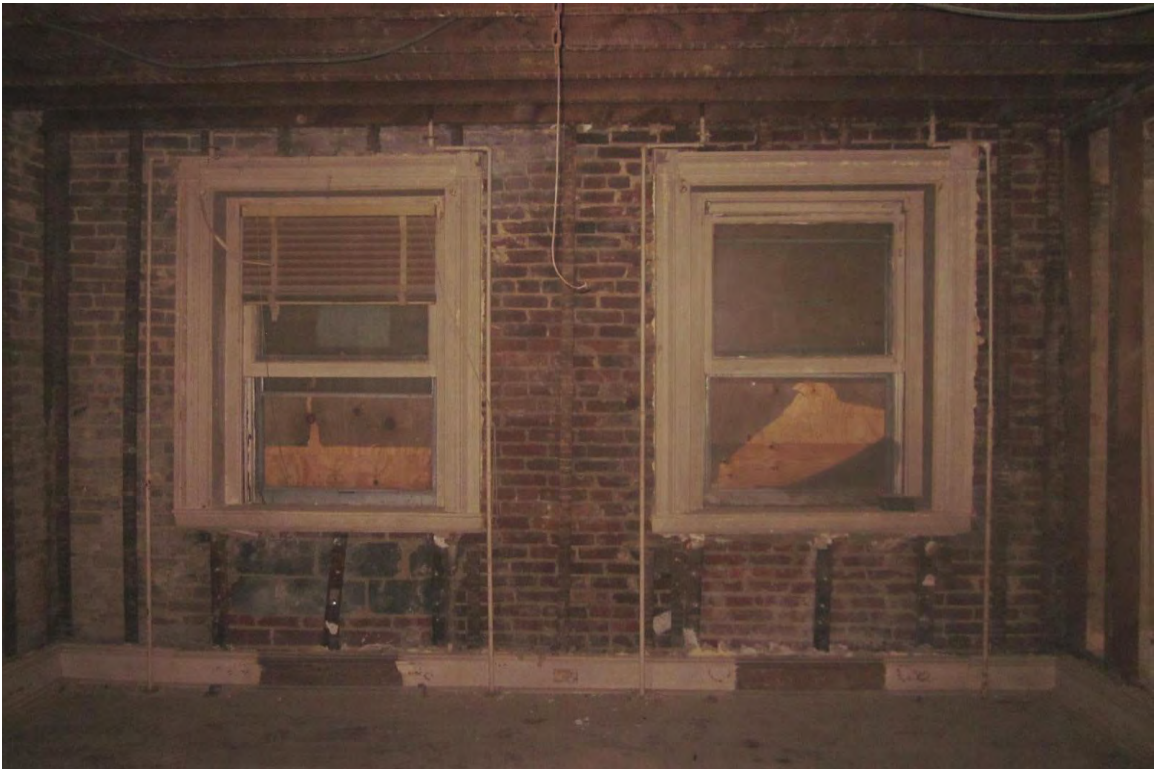
Photo 7.3 Windows, 1/1 original wood windows at Room 3 on the 1 st floor of front façade (see Photo 4.1); Interior Woodwork; Plan (Room 3)
