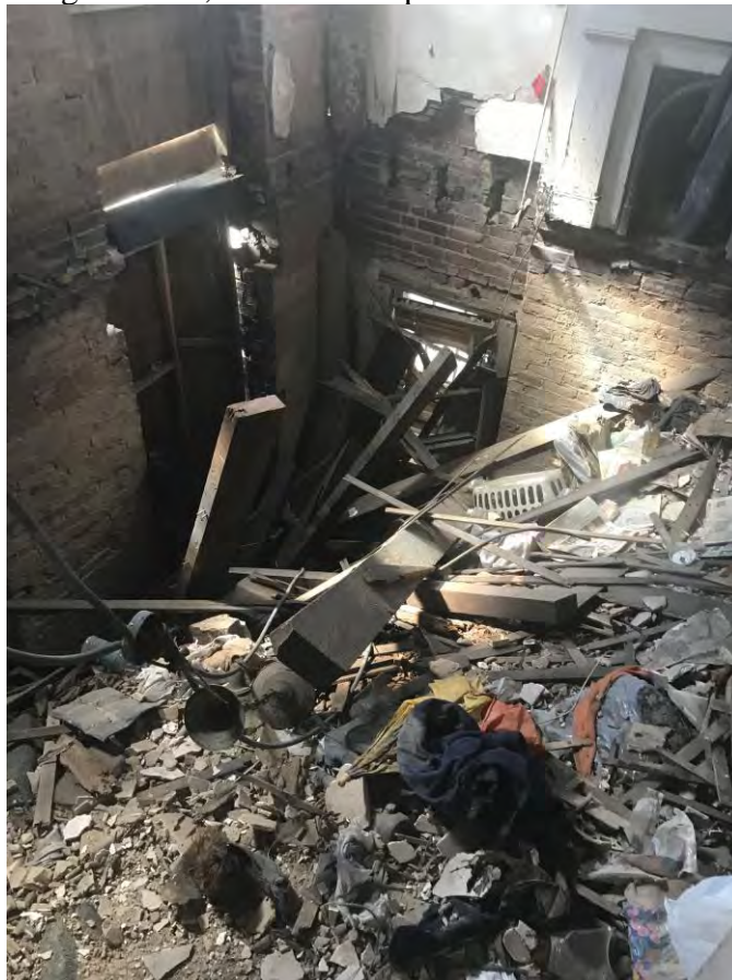
Photo 10.4, Wall and Ceiling Finishes, view of collapsed 2 nd Floor down to collapsed 1 st Floor
