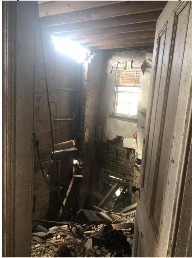
Photo 10.4, Wall and Ceiling Finishes, view of collapsed 2 nd Floor down to collapsed 1 st Floor
