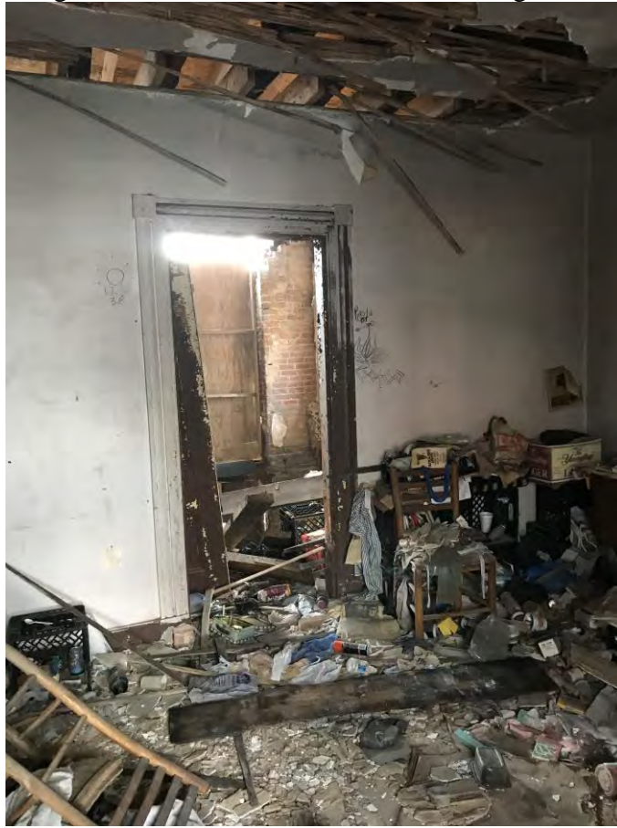
Photo 10.6, Wall and Ceiling Finishes, view of collapsed 2 nd Floor at rear Hall entrance
