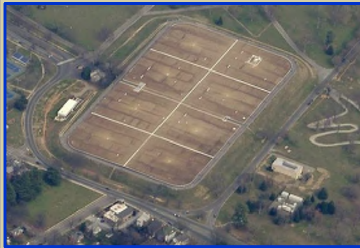
Existing Concrete Roof
