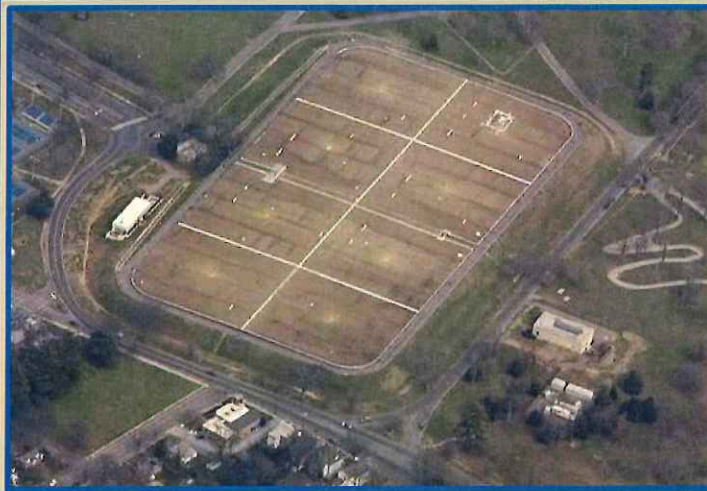
Existing Concrete Roof
