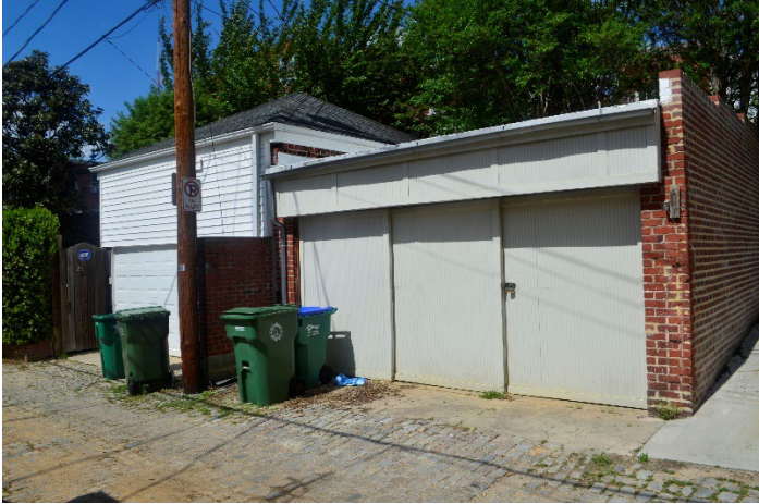
Figure 1. 2915 Monument Avenue garage, along the north side of the alley.
