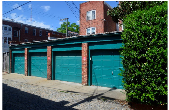
Figure 14. 2923 Monument Avenue garage, located two houses west of 1915 Monument Avenue. This is another example of a low, one-story garage on the same block.
