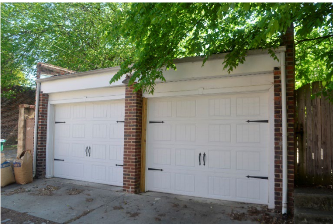
Figure 13. 2908 Park Avenue garage, located on the south side of the alley, southeast of the 2915 Monument Avenue garage.
