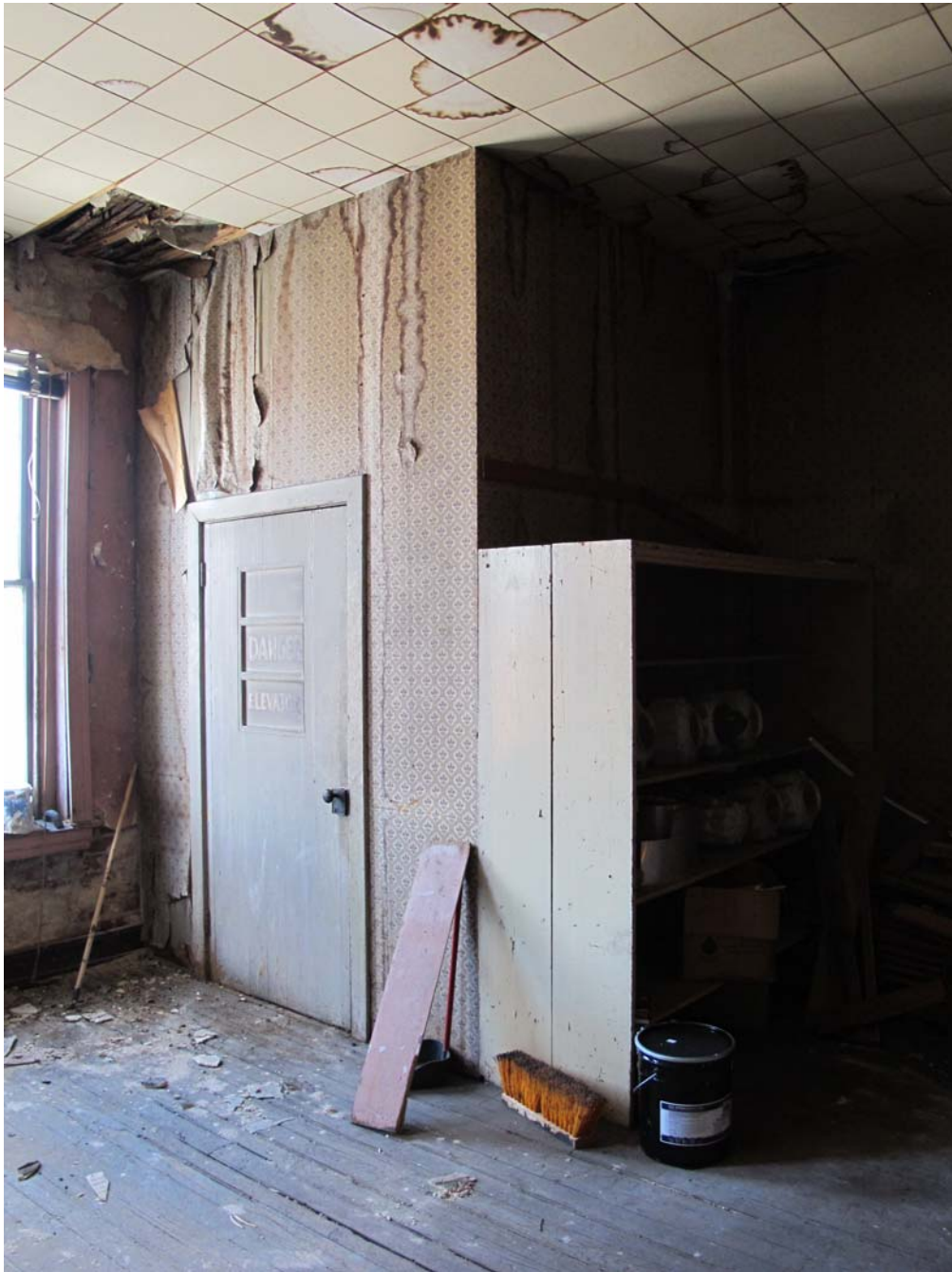
39. Rear elevator enclosure at the 3rd floor.
