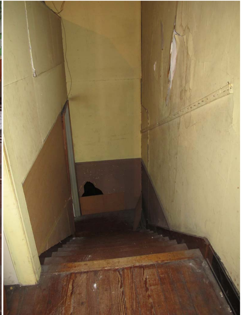
34. Non-historic stair from mezzanine to 2nd floor
