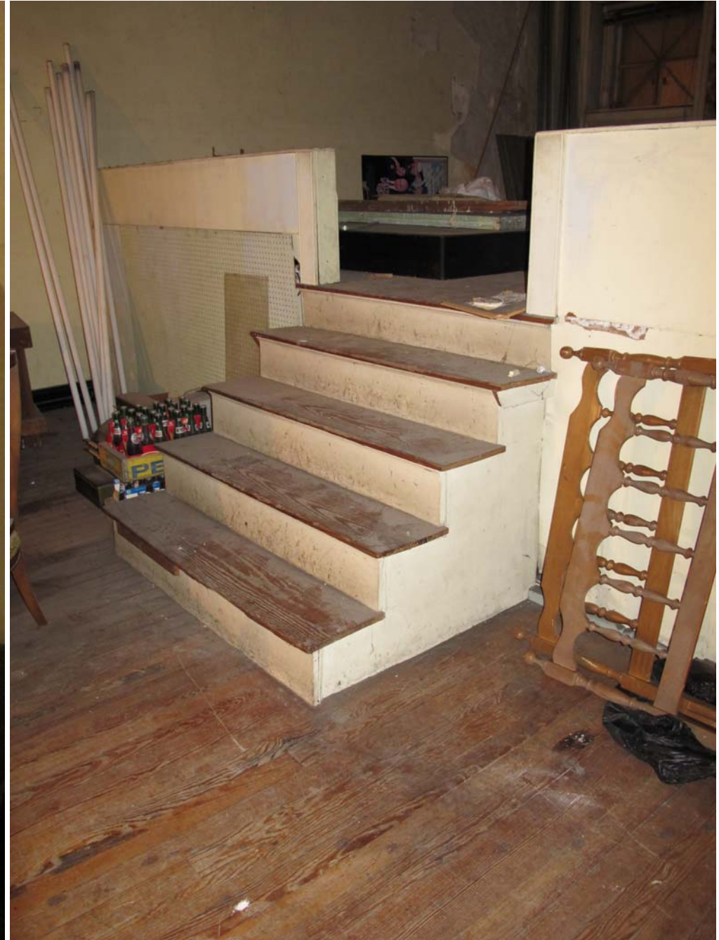
36. Non-historic stair to 2nd floor mezzanine
