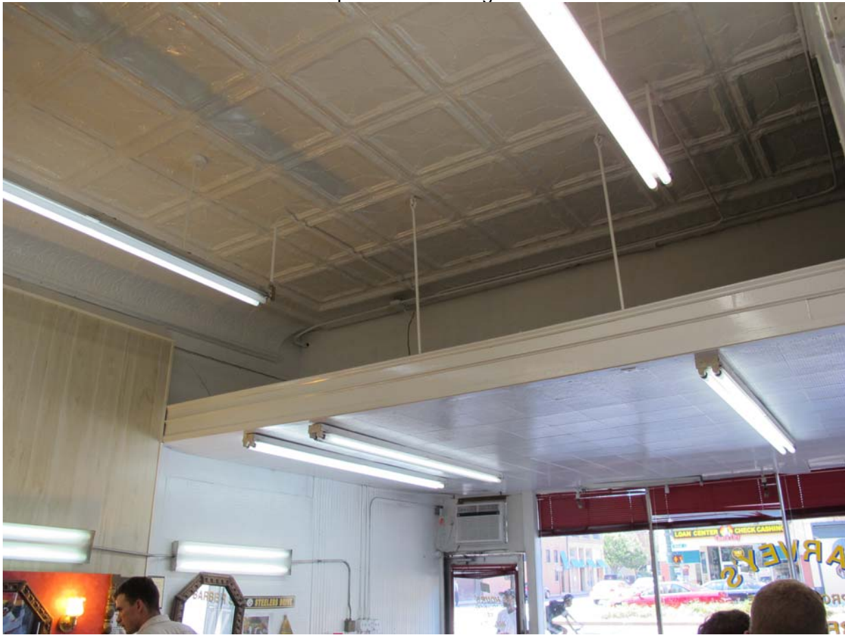
27. Detail of dropped ceiling at 1st floor front
