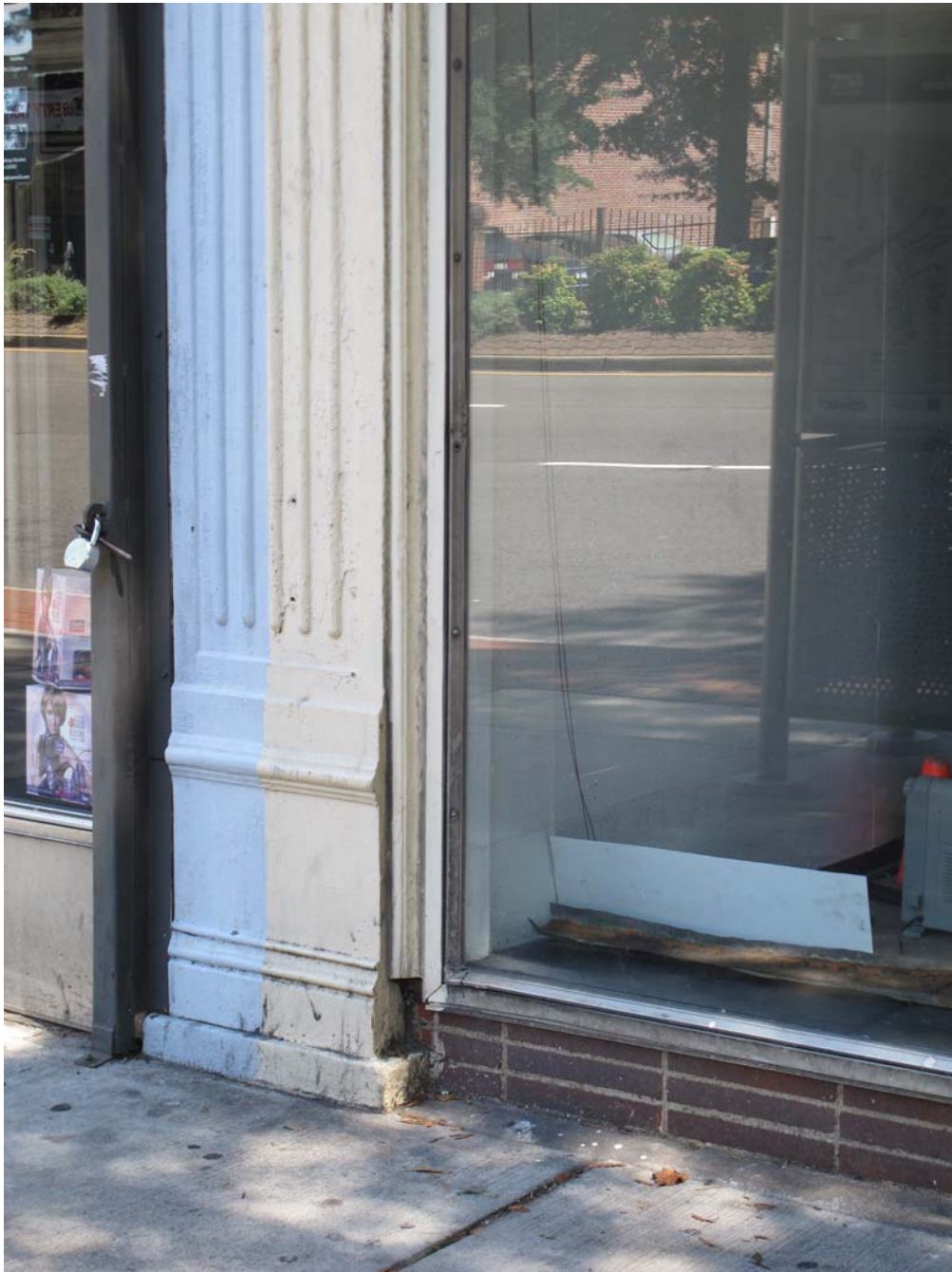
25. Detail of existing storefront bulkhead
