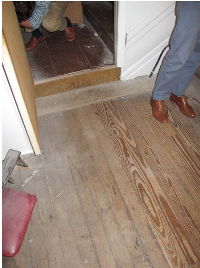
32. Change of flooring at mezzanine extension. Non-historic stair landing
