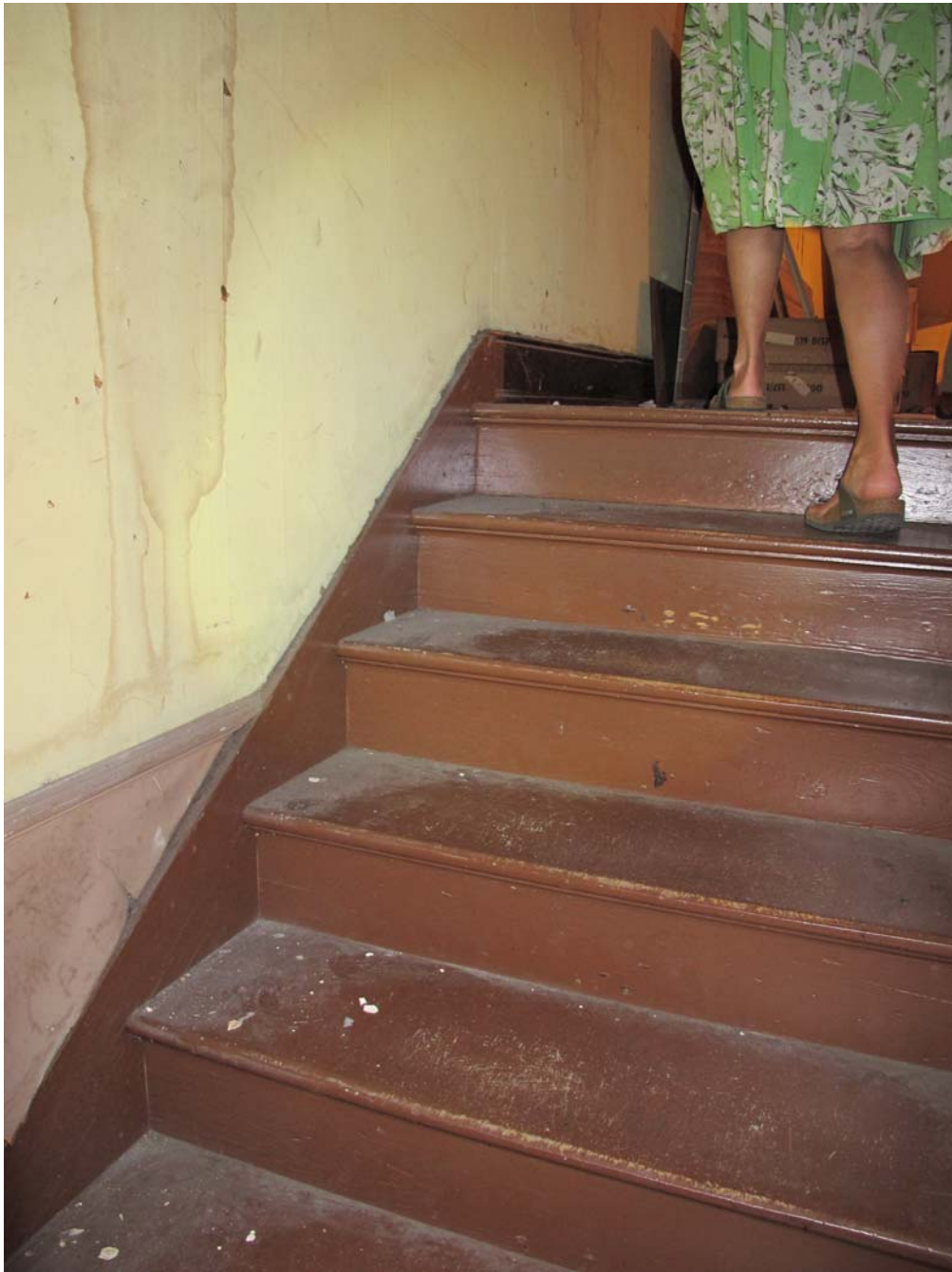
33. Non-historic stair from mezzanine to 2nd floor
