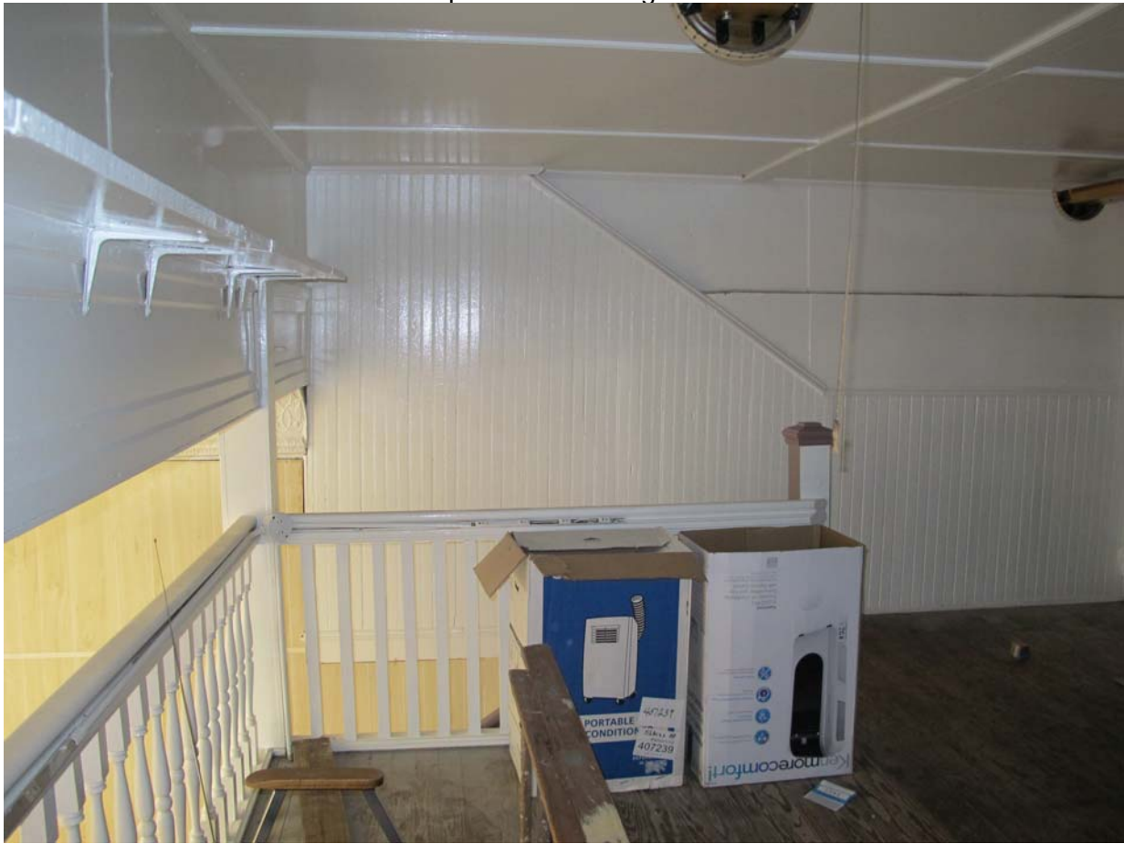
31. Detail of mezzanine. Note former stair rail
