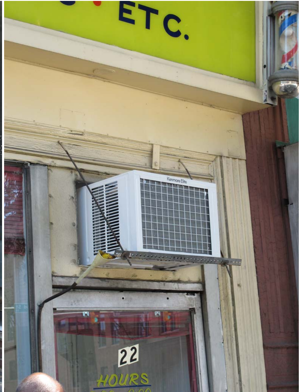
26. Detail of non-historic storefront entry
