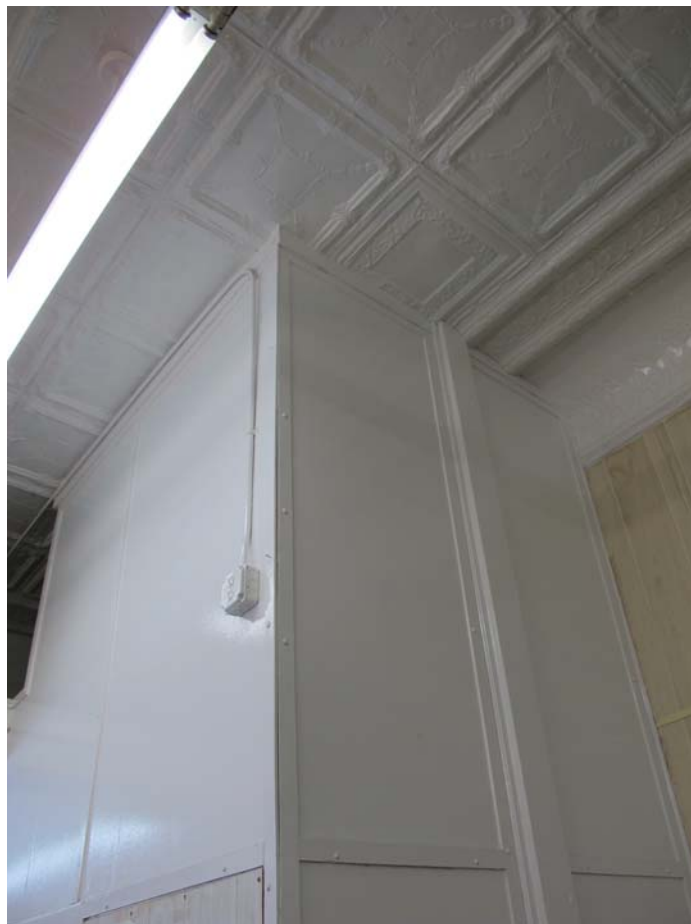
28. Detail of non-historic elevator enclosure
