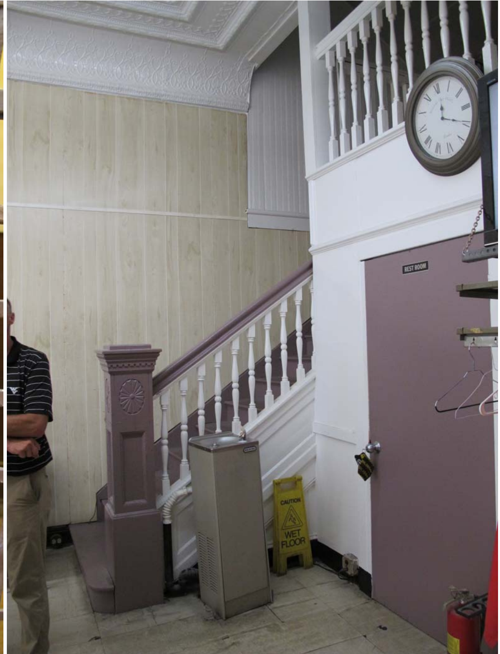
30. Relocated stair to mezzanine
