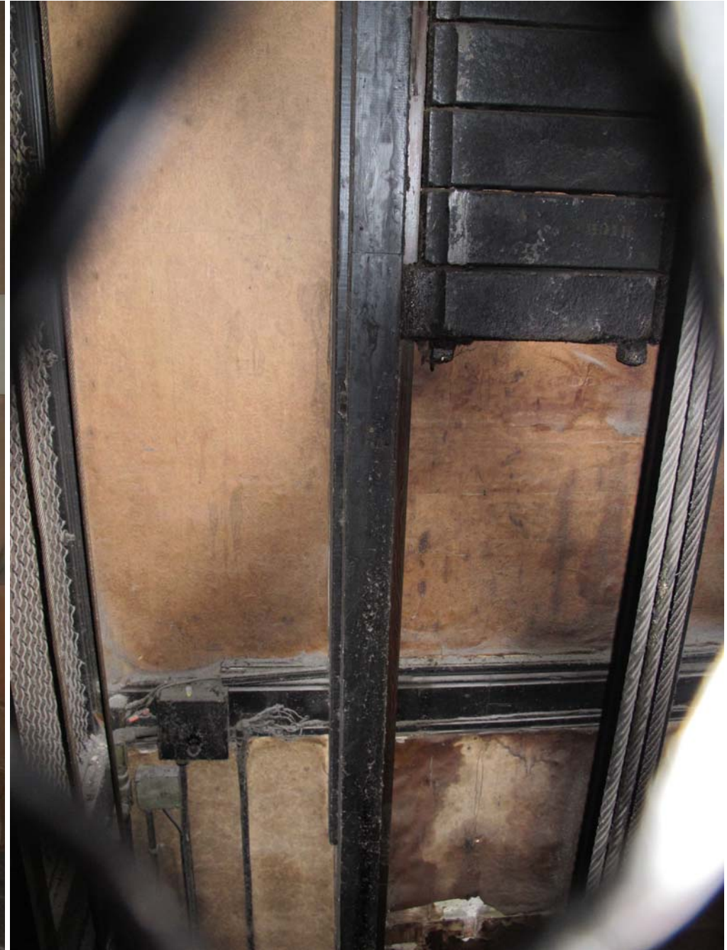
38. Detail within front elevator shaft at 2nd fl
