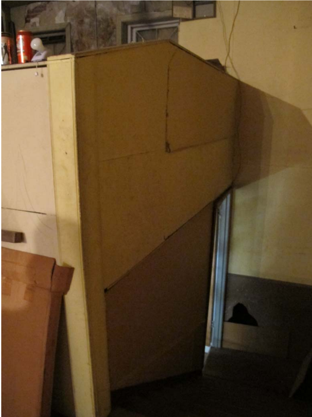
35. Non-historic stair enclosure at 2nd floor mezzanine
