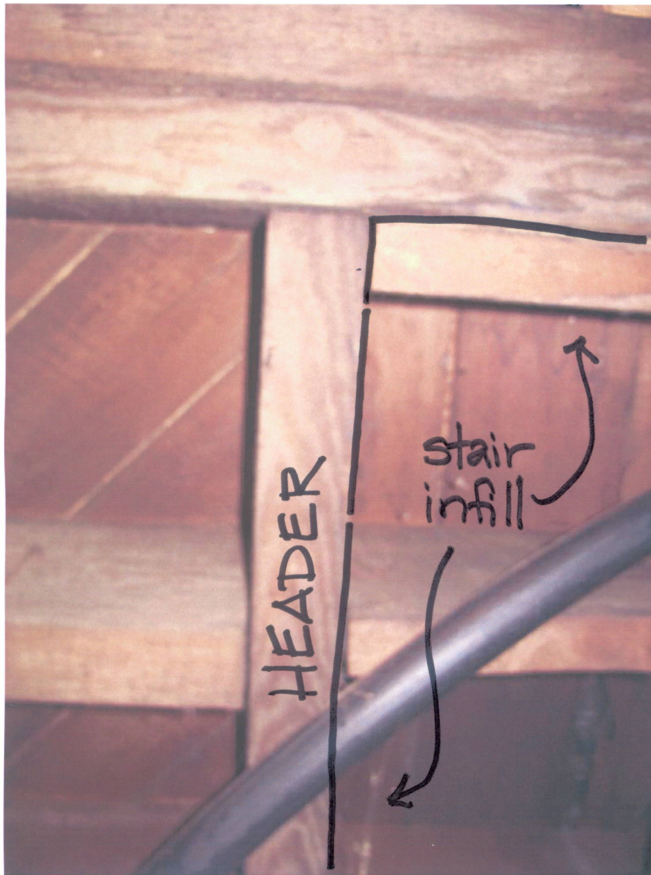
41. Detail of original stair opening between basement and 1st floors
