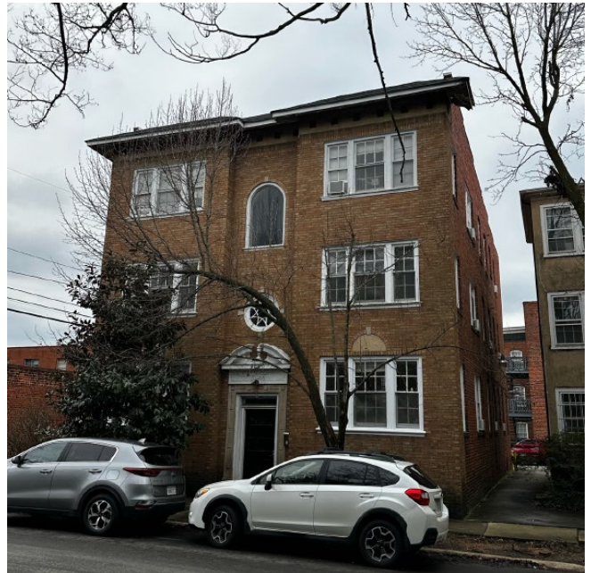
Figure 4. Existing roof condition, asphalt shingles
