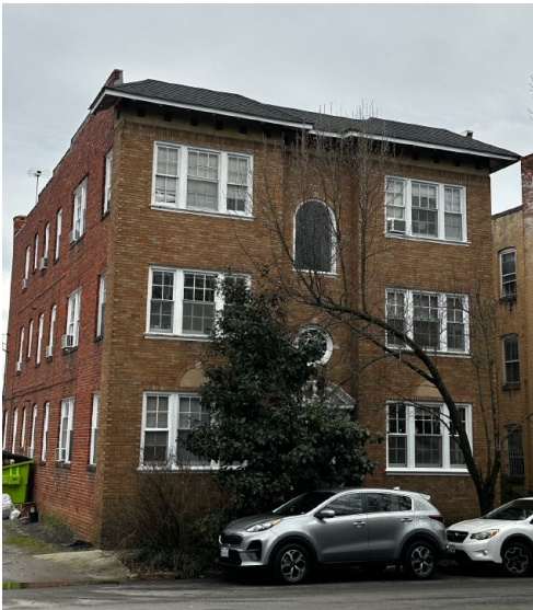
Figure 3. Existing roof condition, asphalt shingles
