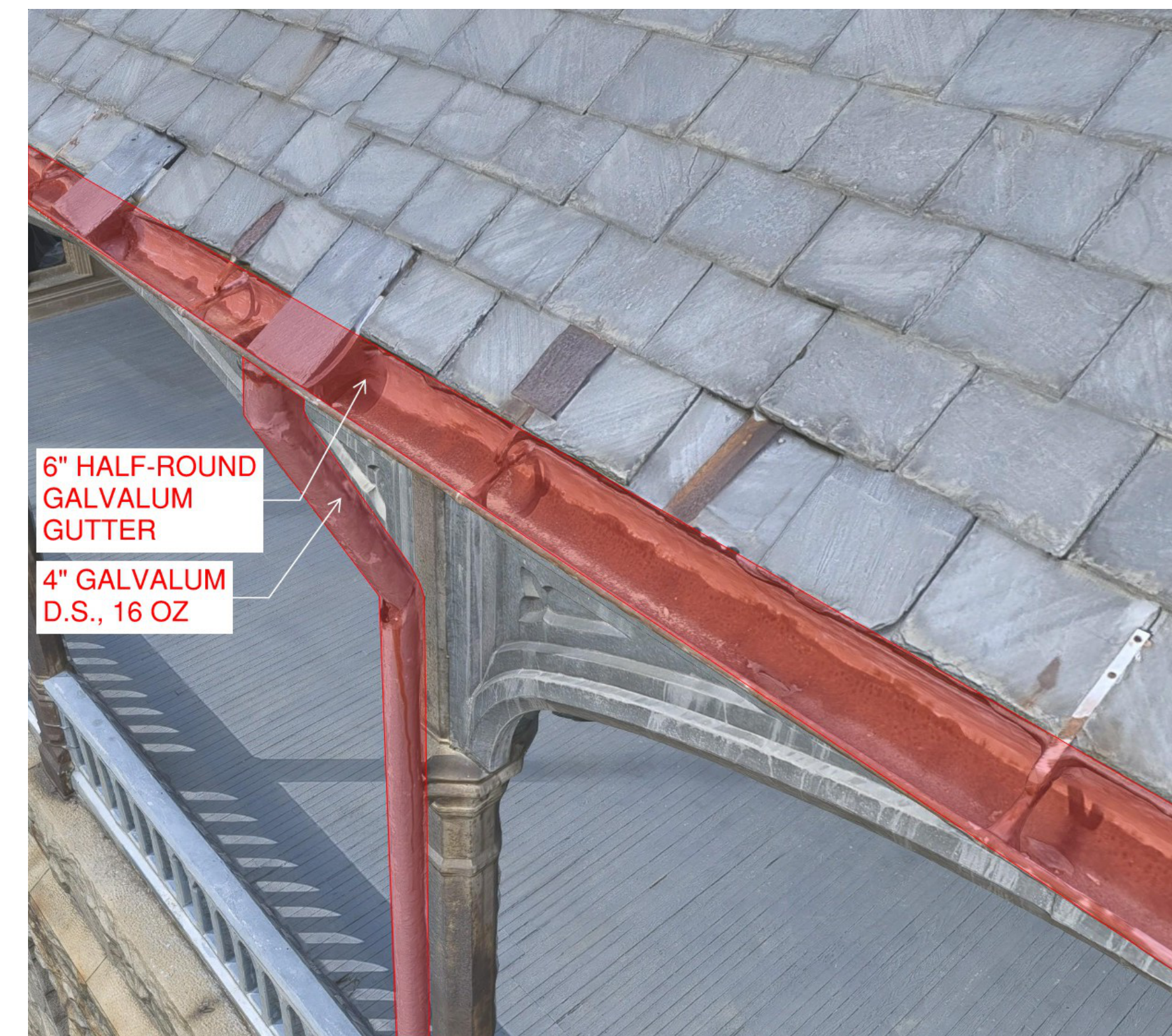
J11 WALL SECTION - EAVE @ SOUTH PROMENADE A010 1" = 1'-0" REFERRED FROM:A009
