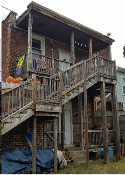
Figure 7. 3105 East Marshall Street, rear elevation.
